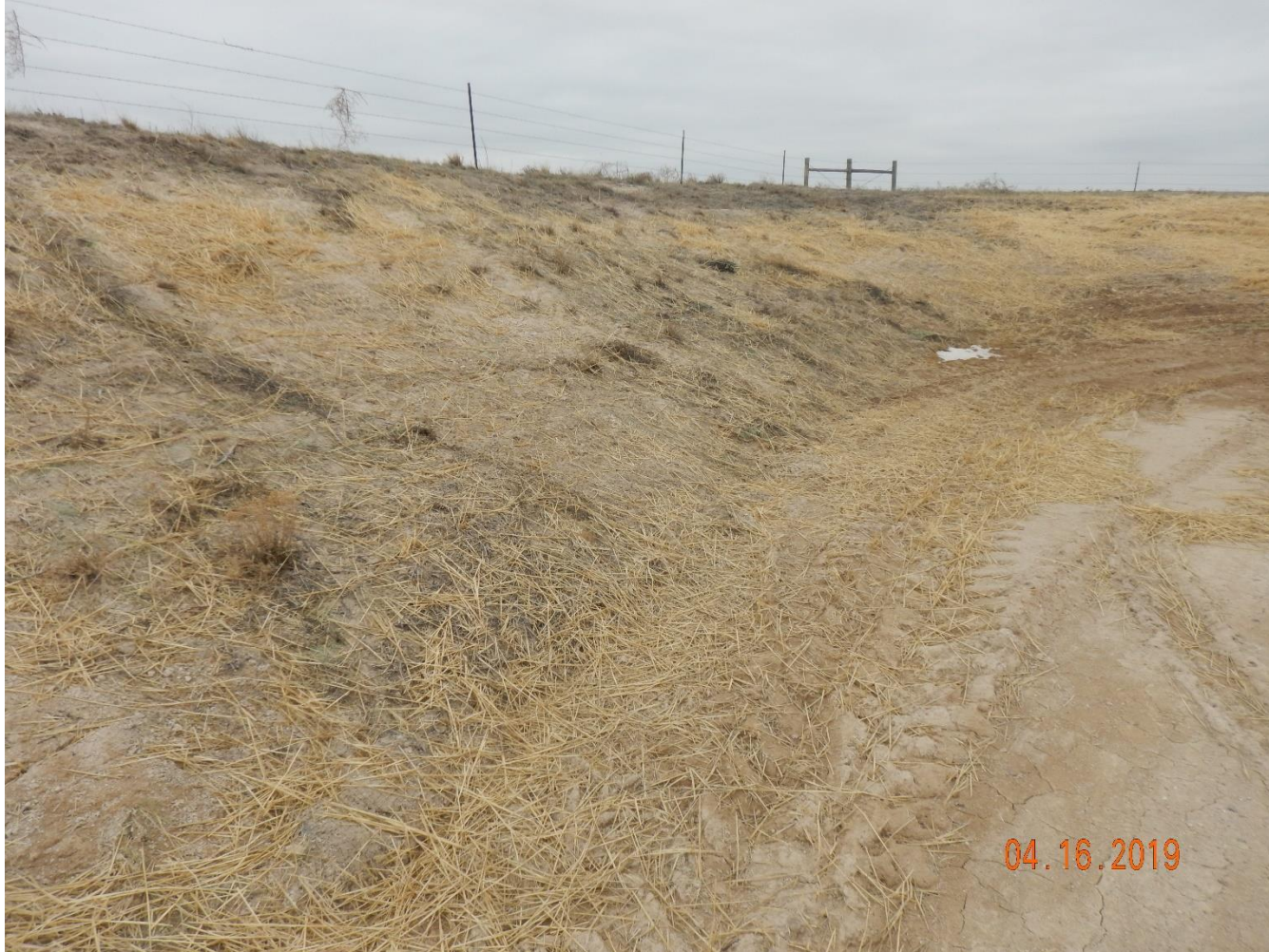
Photo 4: Photo taken from the south end of the location, facing west. Photo slopes appear to have been seeded and mulched.
