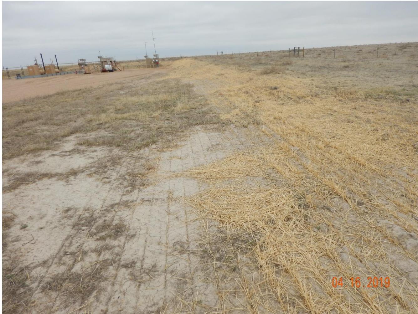
Photo 3: Photo taken from the west interim area of the location, facing south. Photo slopes appear to have been seeded and mulched.
