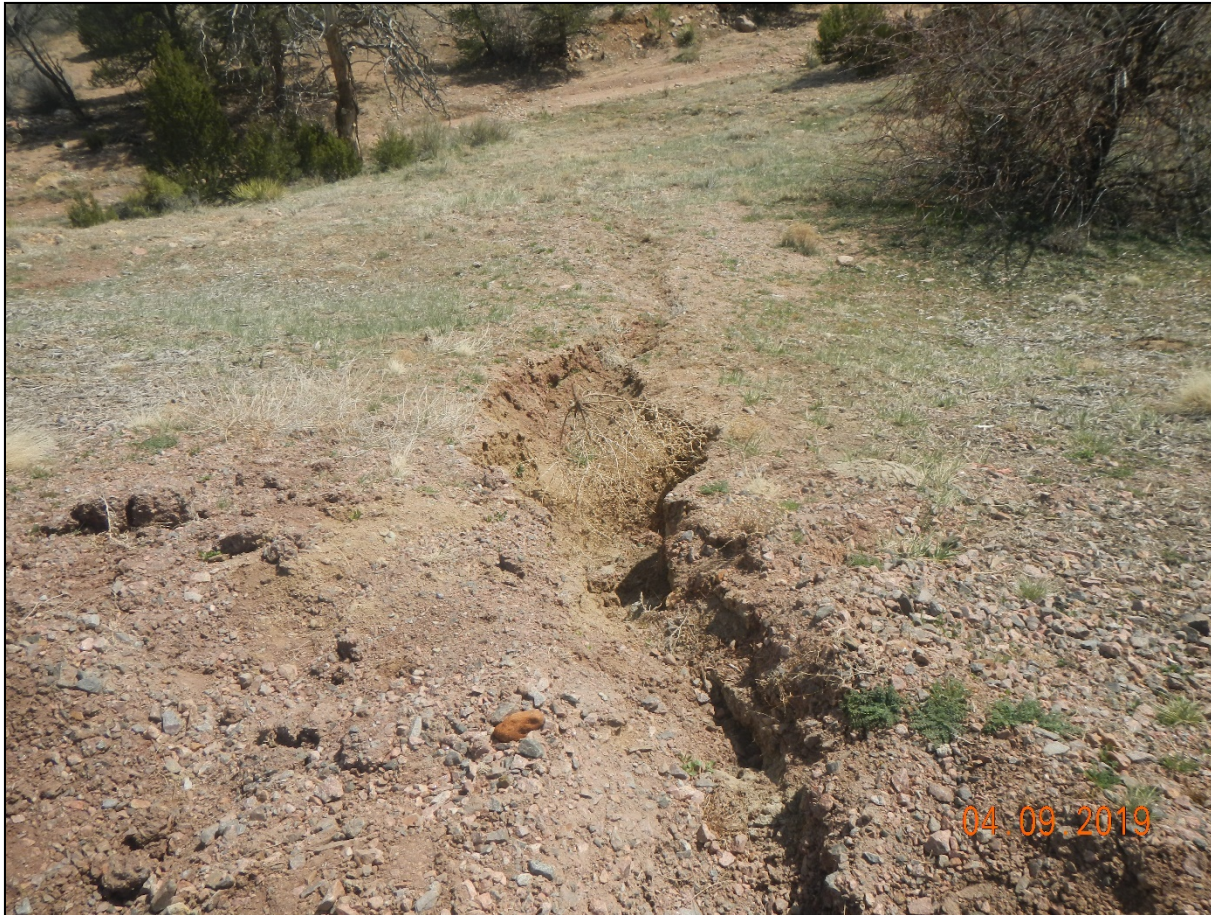
Photo 3. Erosion channel has not been repaired at the east side of the location.
