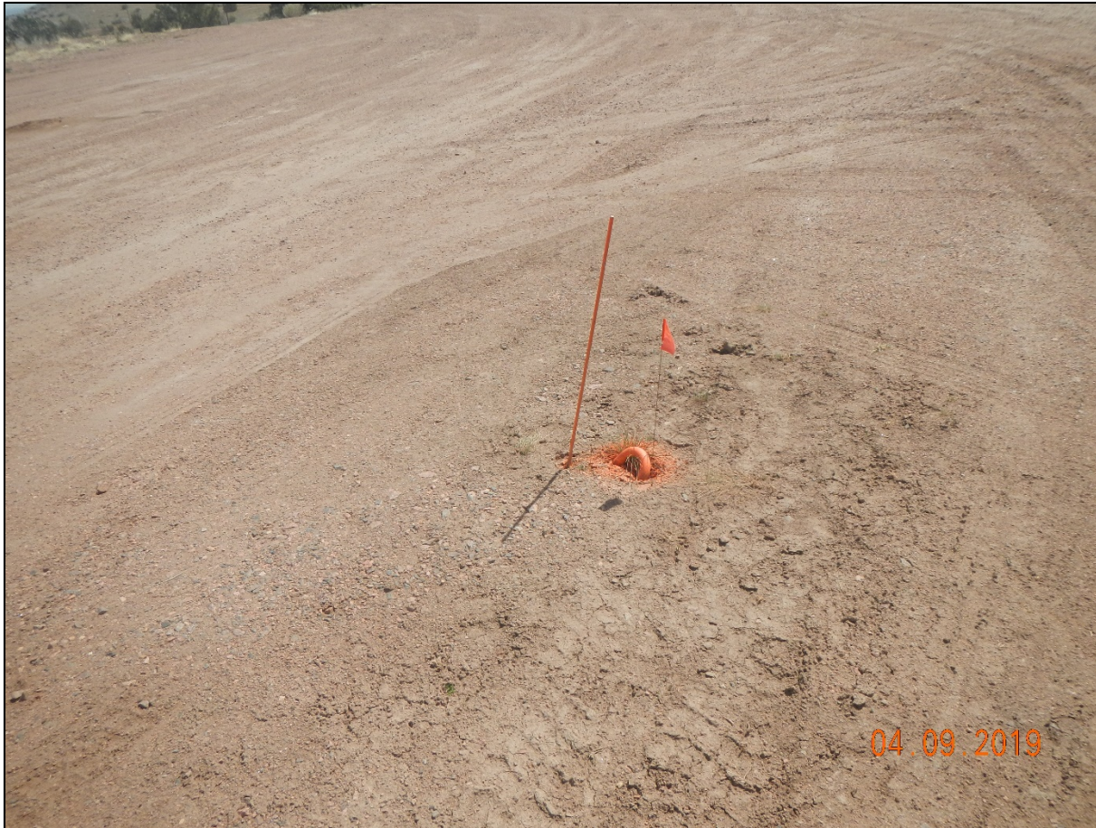
Photo 2. Guyline anchors have been marked, however markers should be not less than 4ft. In height.
