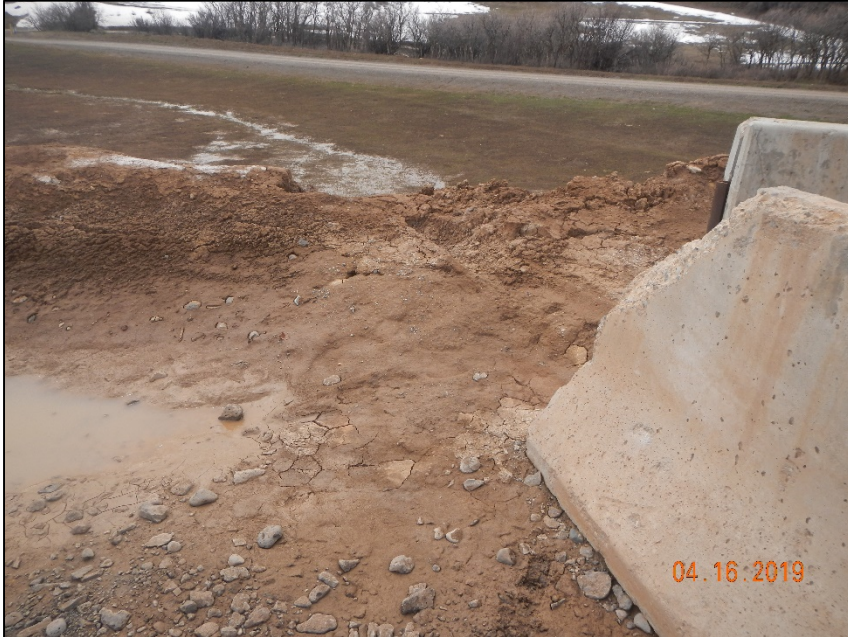
Berm has evidence of erosion and needs repaired
