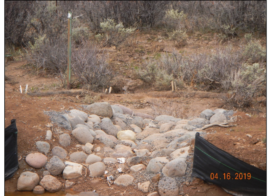
Sediment moving over the top of wattle. In need of maintenance.
