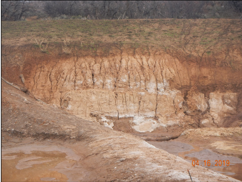
Heavy erosion of hill side do to no stabilization
