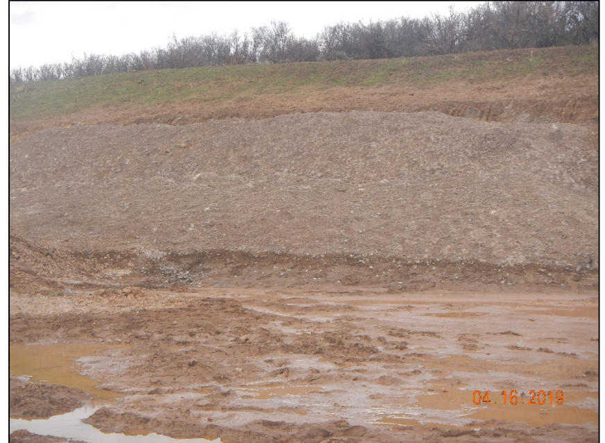
No Berm around soil pile
