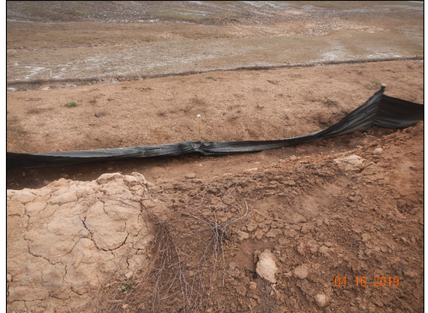
Silt fence BMP needs maintenance
