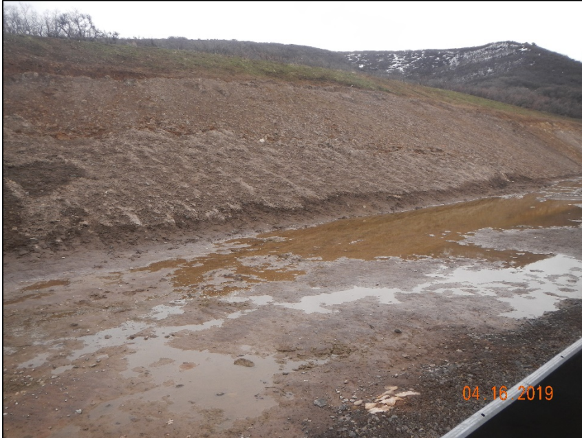
No Berm around soil pile
