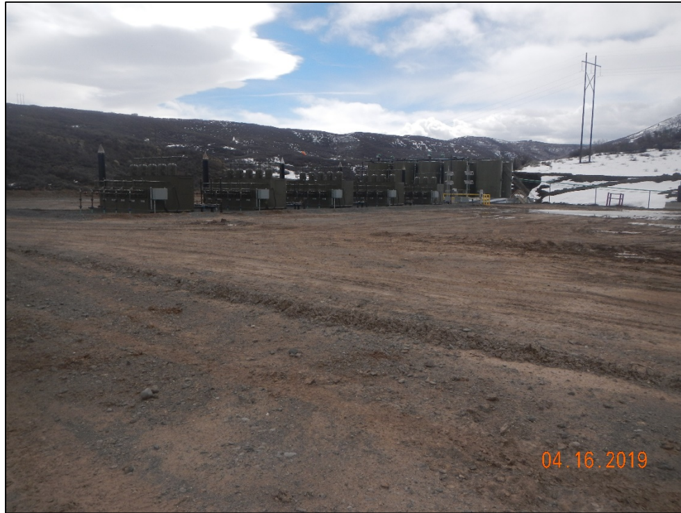
Photo of location
