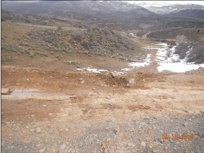
Erosion through berm,
