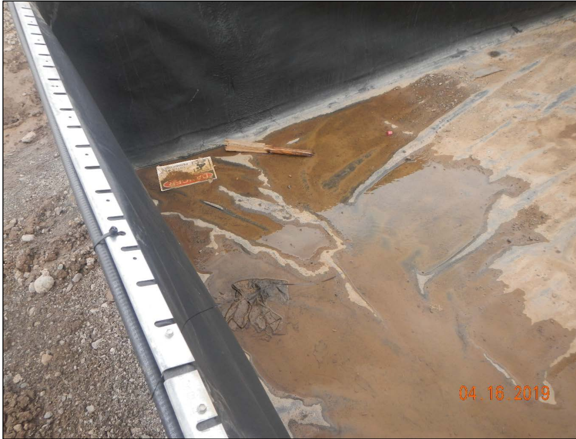
Trash inside tank containment
