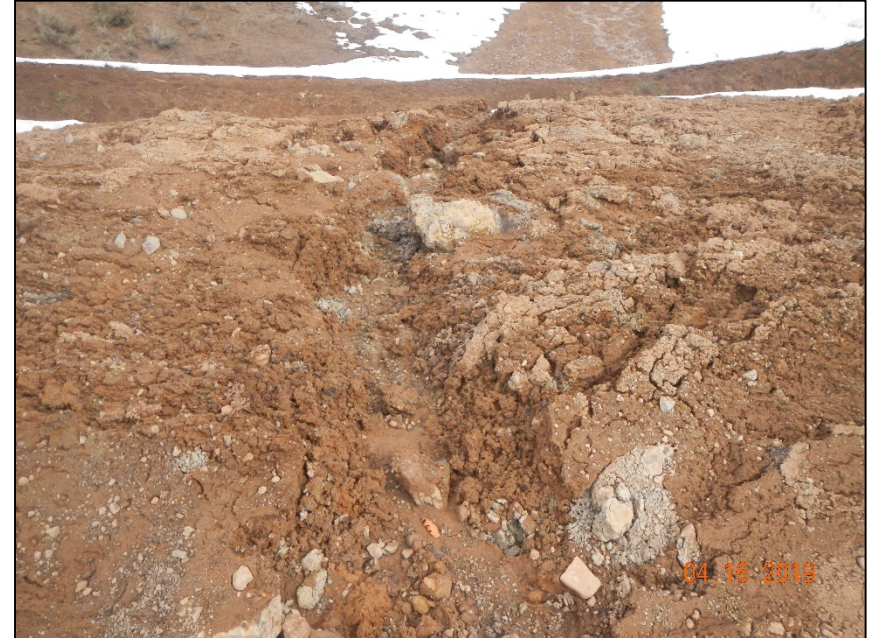
Close up of erosion through berm
