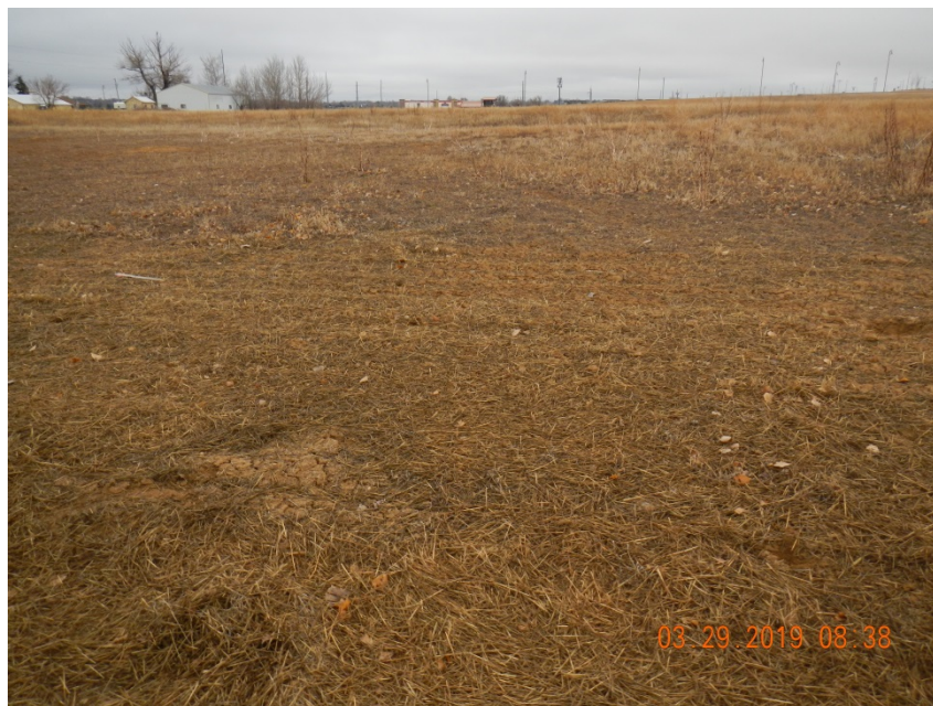
Photo 6. Photo taken from the location, facing Southeast. Appears reclamation activities have recently been performed with the evidence of drill rows and straw crimped mulch.
