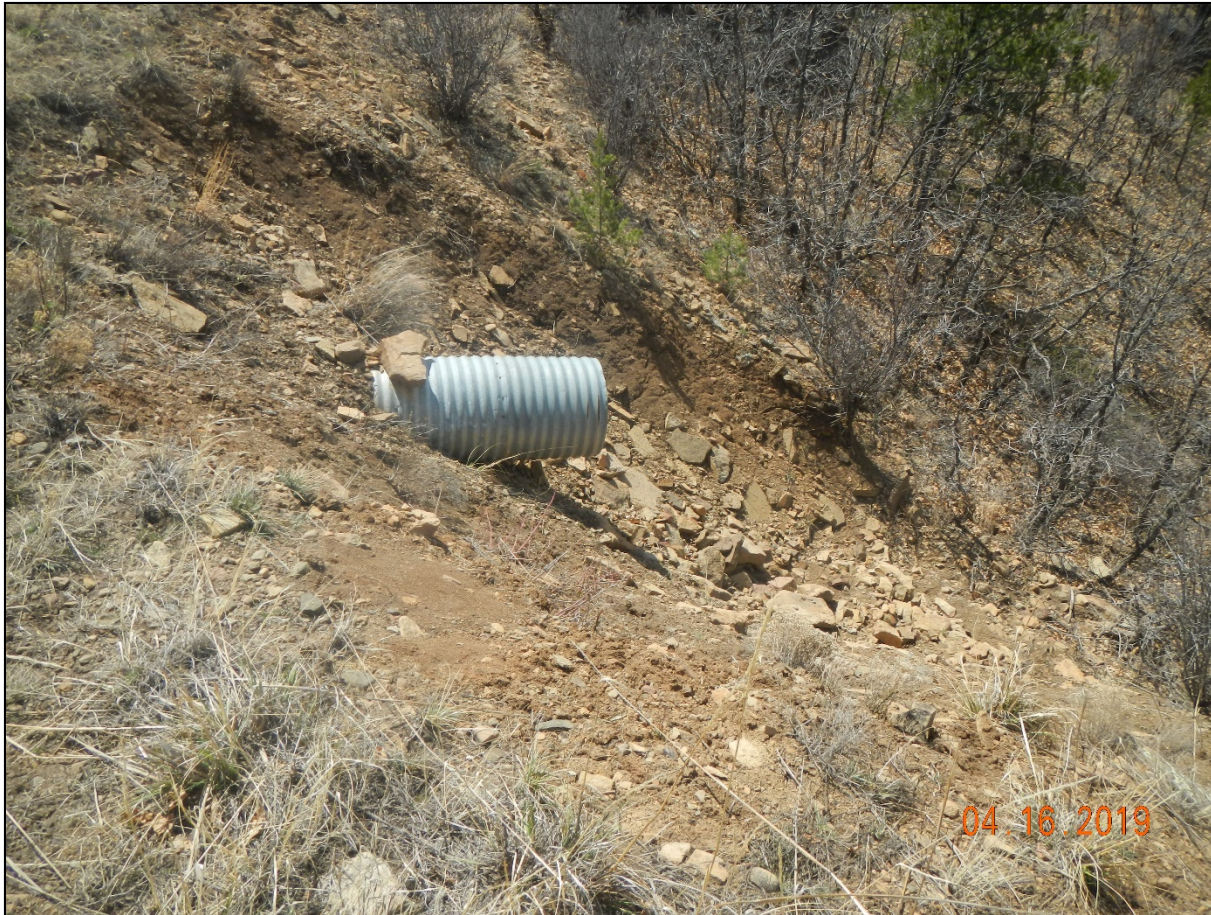
Photo 4. Culvert remains along the road. Erosion is occurring around the outlet.
