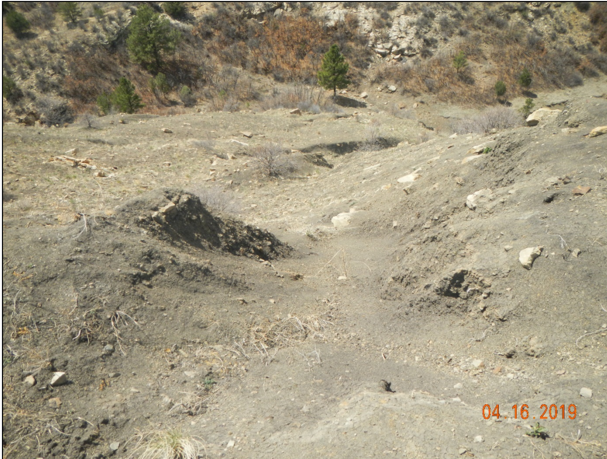
Photo 7. Facing down the fill slope shows signs of erosion.
