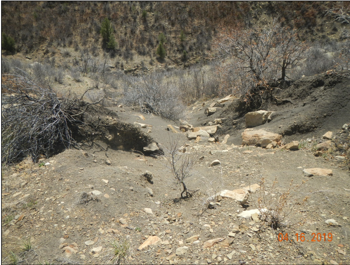
Photo 9. There is significant signs of erosion off the southeast fill slope.
