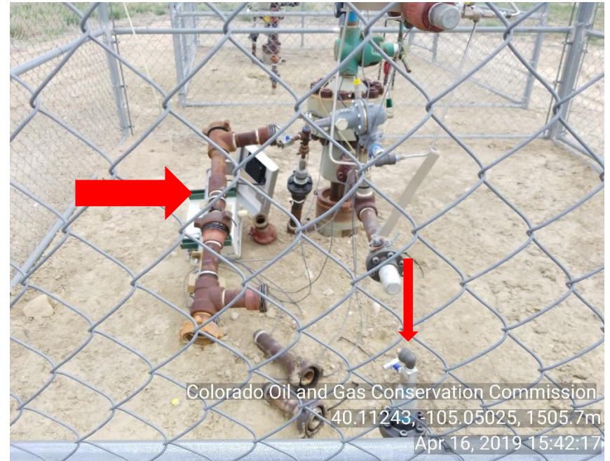
Photo 2 2" piping from WH to flow line disconnected and laying on ground. Unused equipment and unmarked, unused and not LOTO riser.
