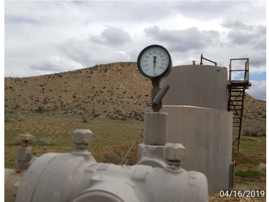
Photo 2. Tubing casing pressure.
