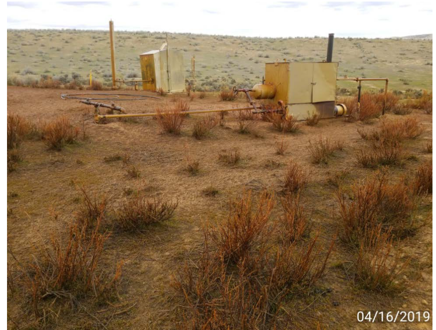
Photo 6. Hydrocarbon stained brush and ground.
