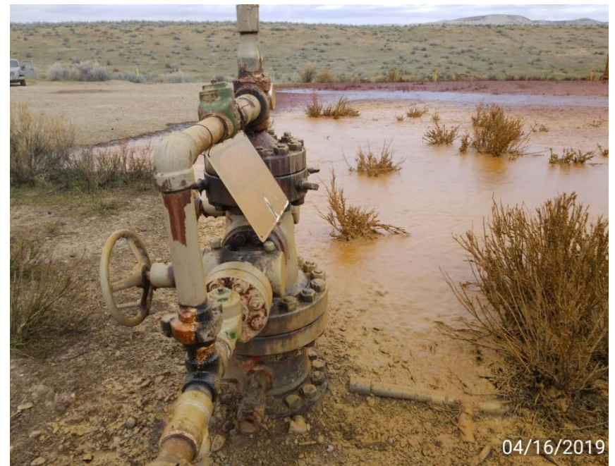
Photo 4. Well head looking northwest.
