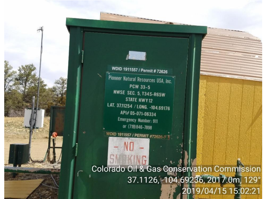
PHOTO 2: METER HOUSE/WELL SIGN
