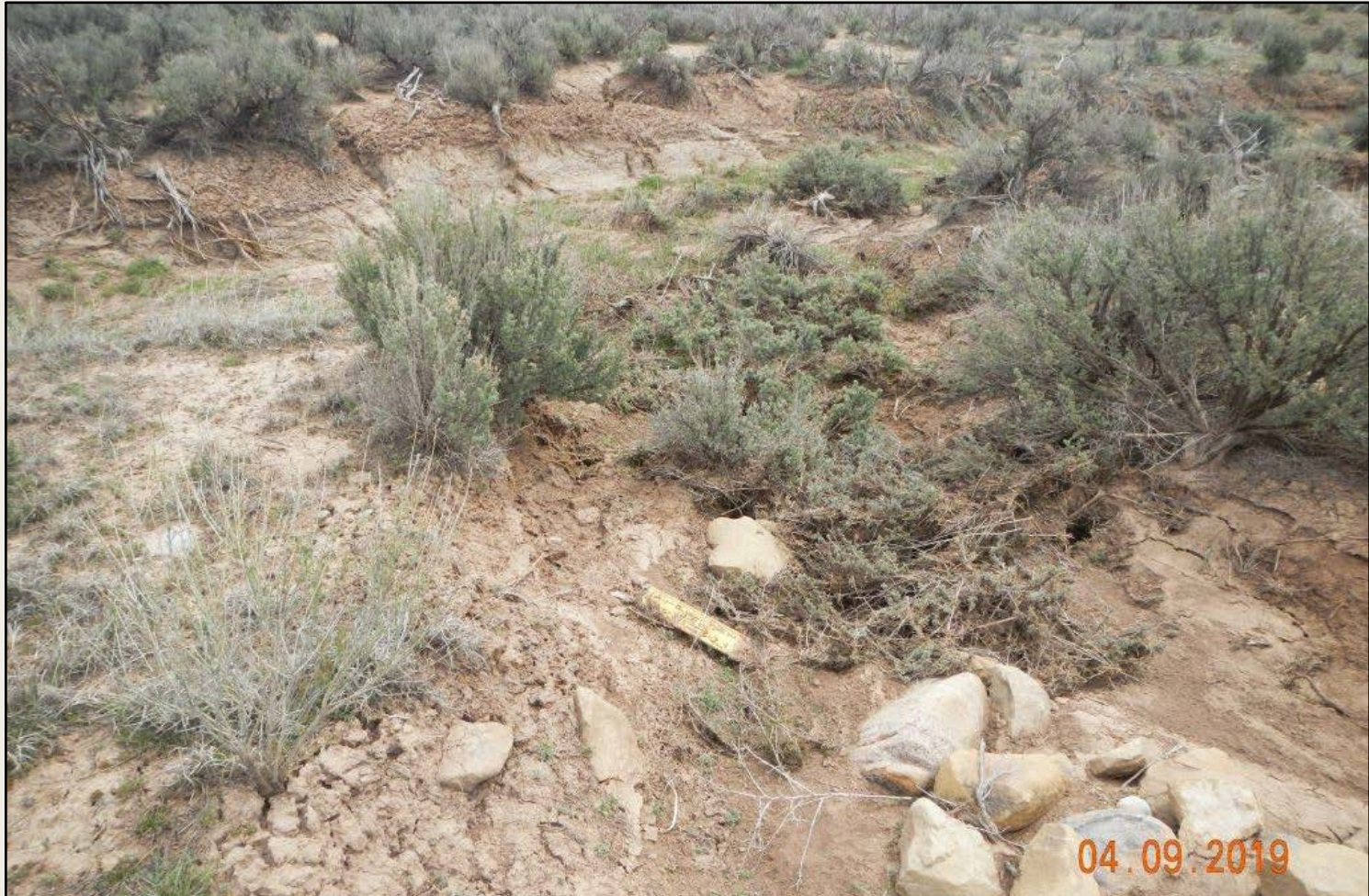
Photo 6. View of erosional scouring from stormwater flows that appear to have breached the access road and are eroding down slope.
