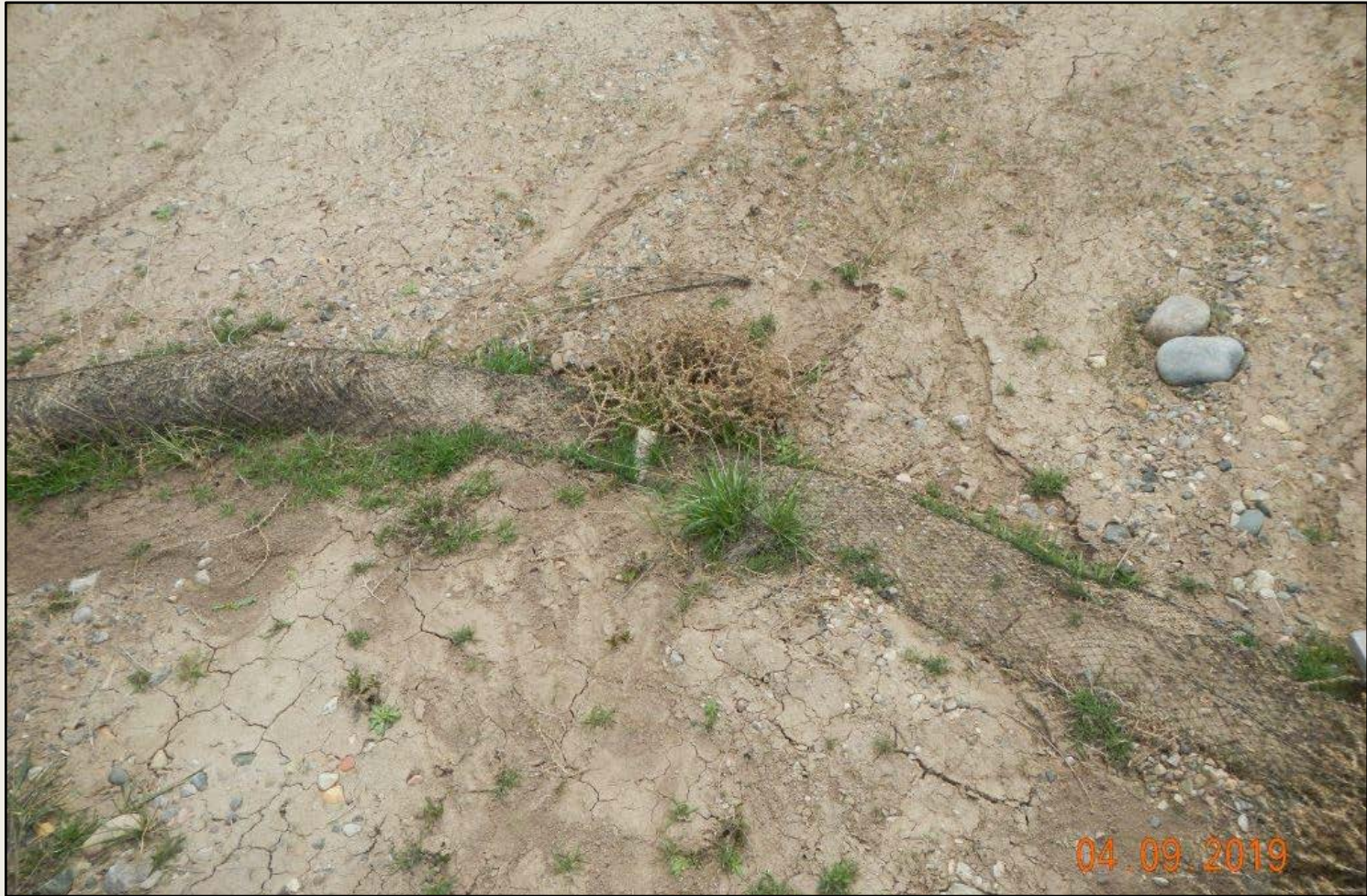
Photo 5. View of wattles no longer functioning within the eastern project area. This stormwater control is not sufficient to manage erosion within this area.
