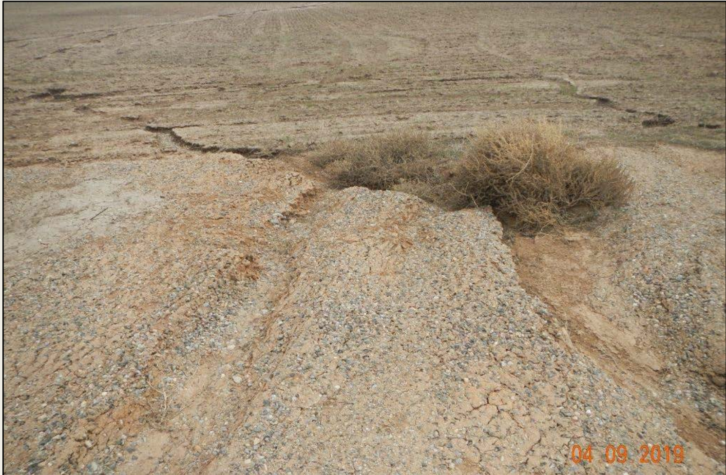
Photo 4. View of erosional channeling and sediment discharge within the eastern project area, facing eastward toward the surrounding cultivated field.
