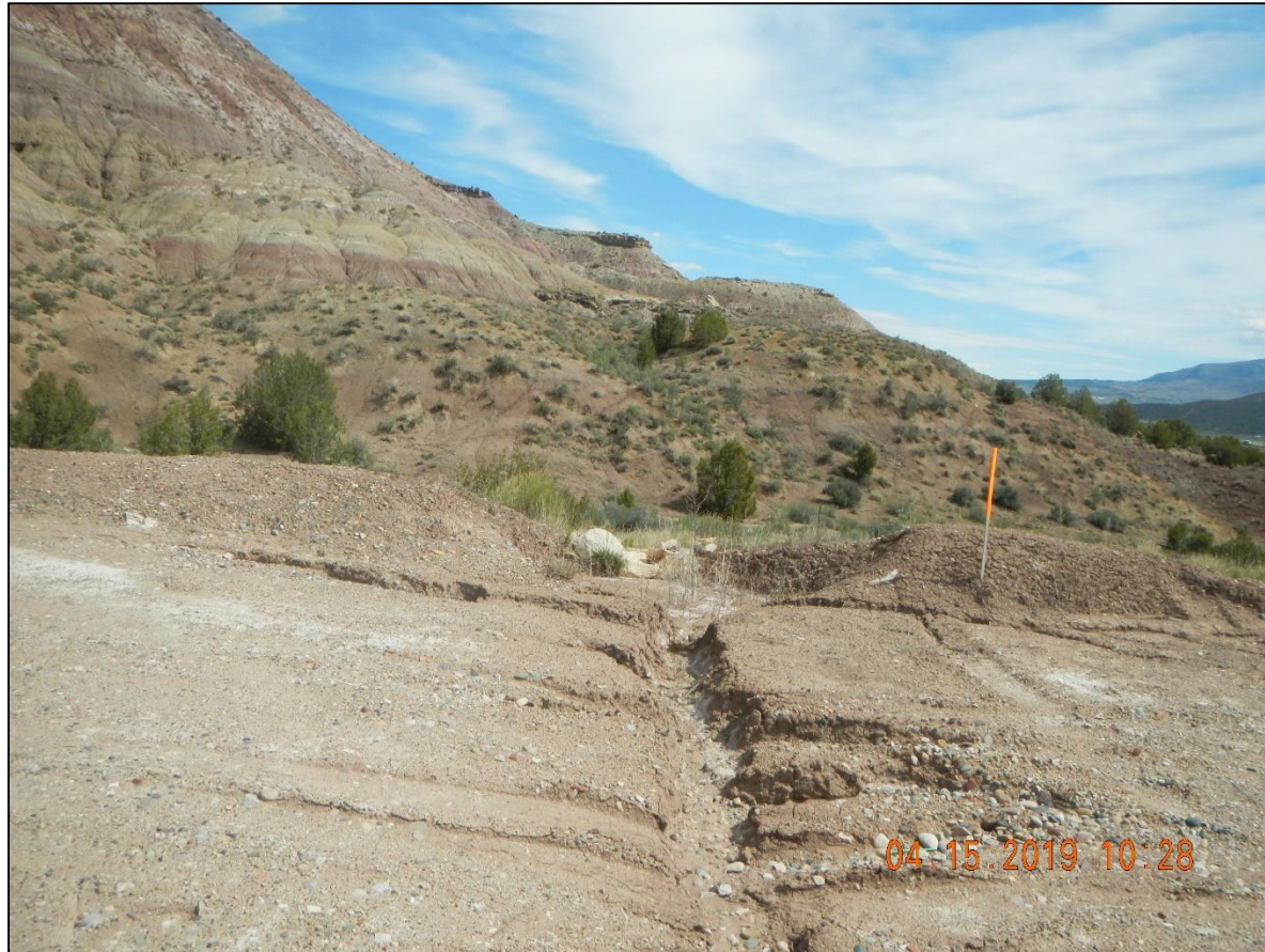
Erosion of location in drainage into check dam.
