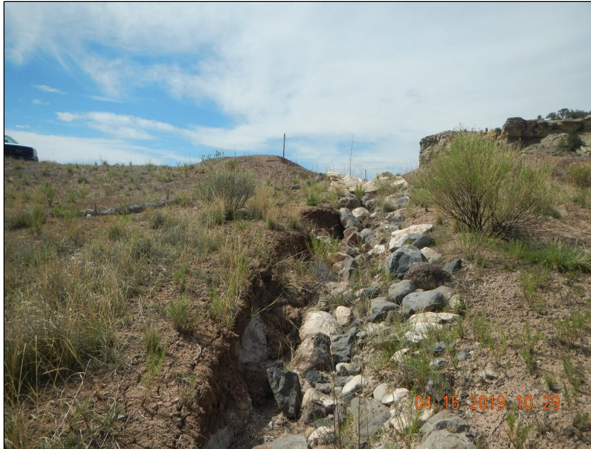
Washing of ditch from check dam.
