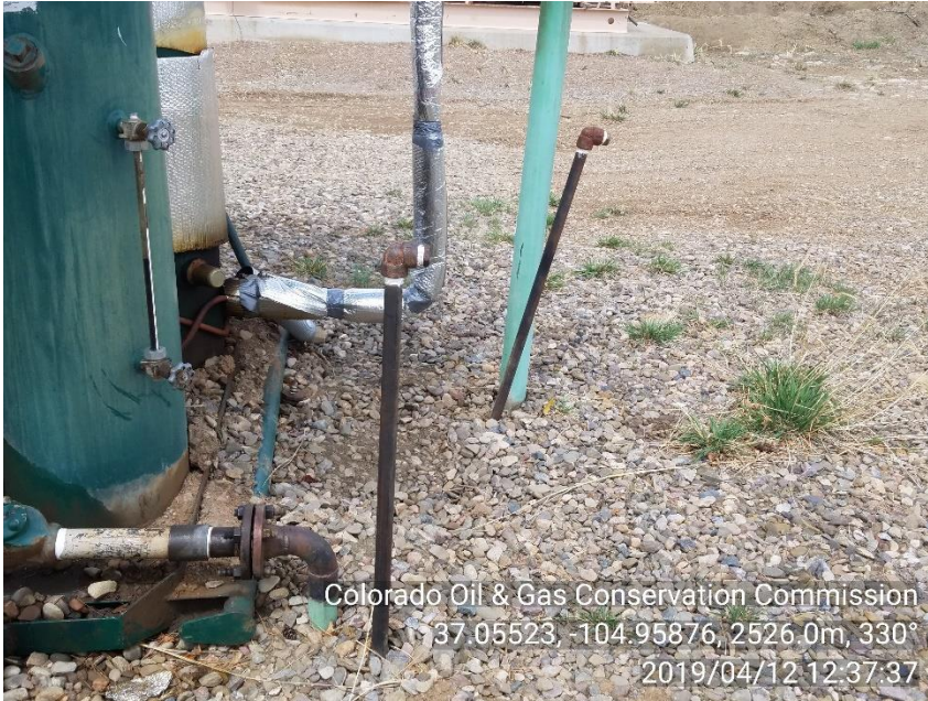
PHOTO 5: TWO UNMARKED 1" RISERS NORTHEAST SIDE OF COMPRESSOR SKID.
