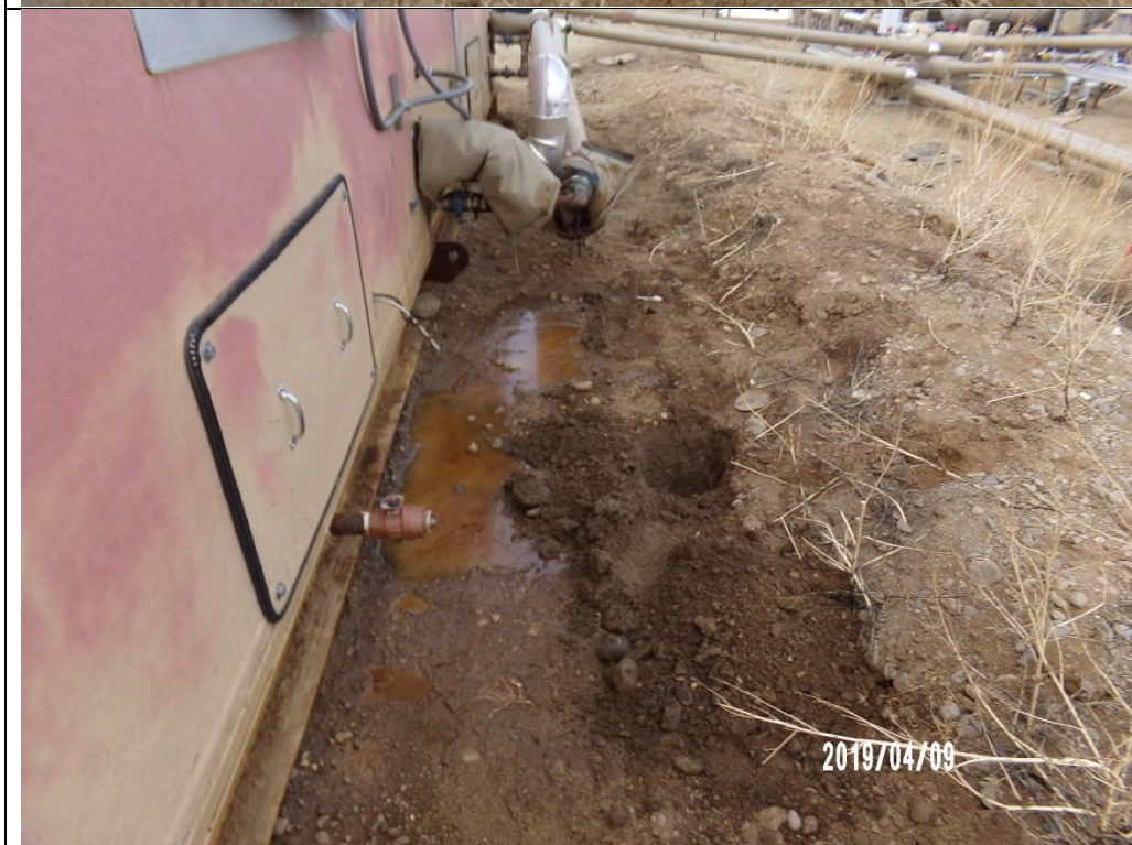
Photo 4: Close up view of spill area after hydrovac removal of hydrocarbons on surface.
