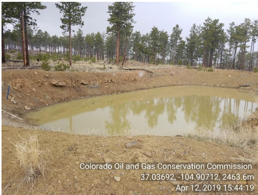
Photo Produced water pit #2
