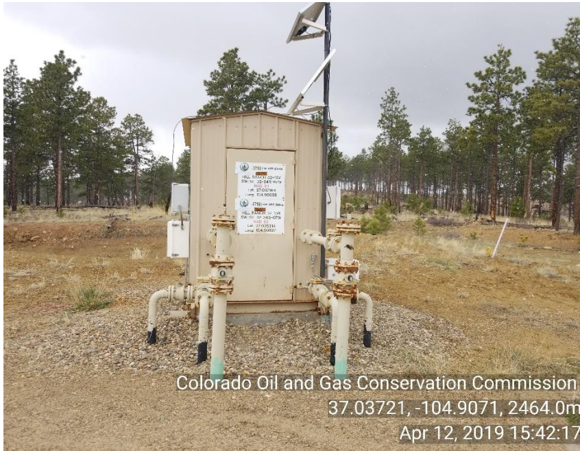
Photo 1 HR#32-15R and HR#32-15V Duel sep/meter house
