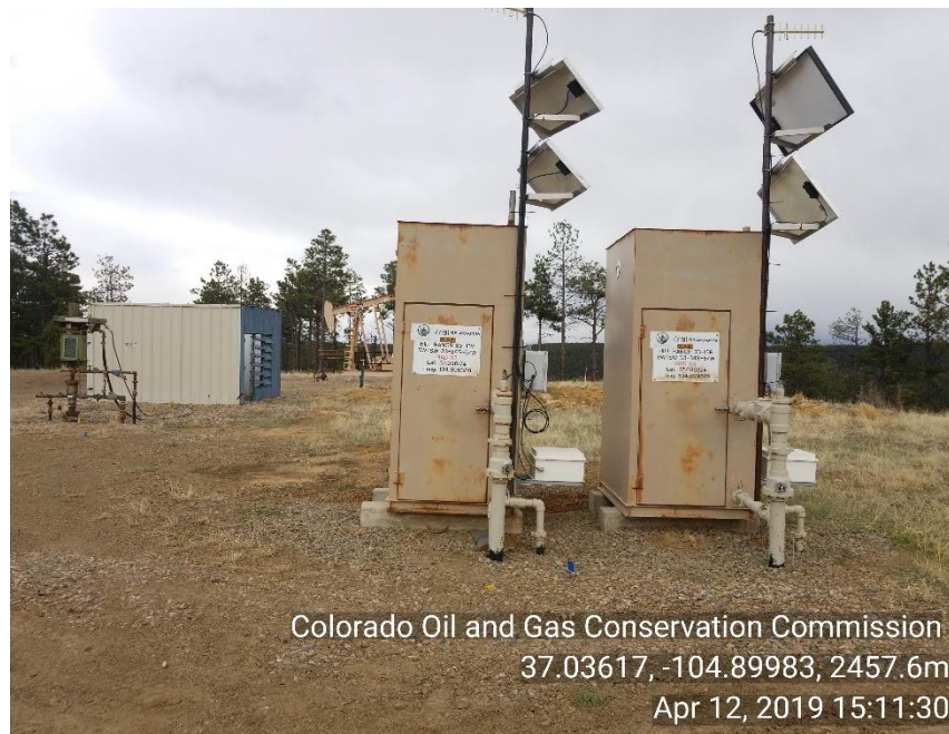
Photo 1 HR#33-13R and HR#33-13V Sep/meter houses
