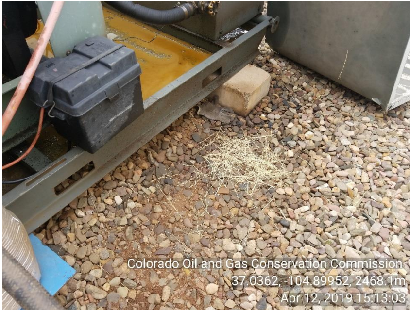
Photo 3 Stained soil around HYD motor skid
