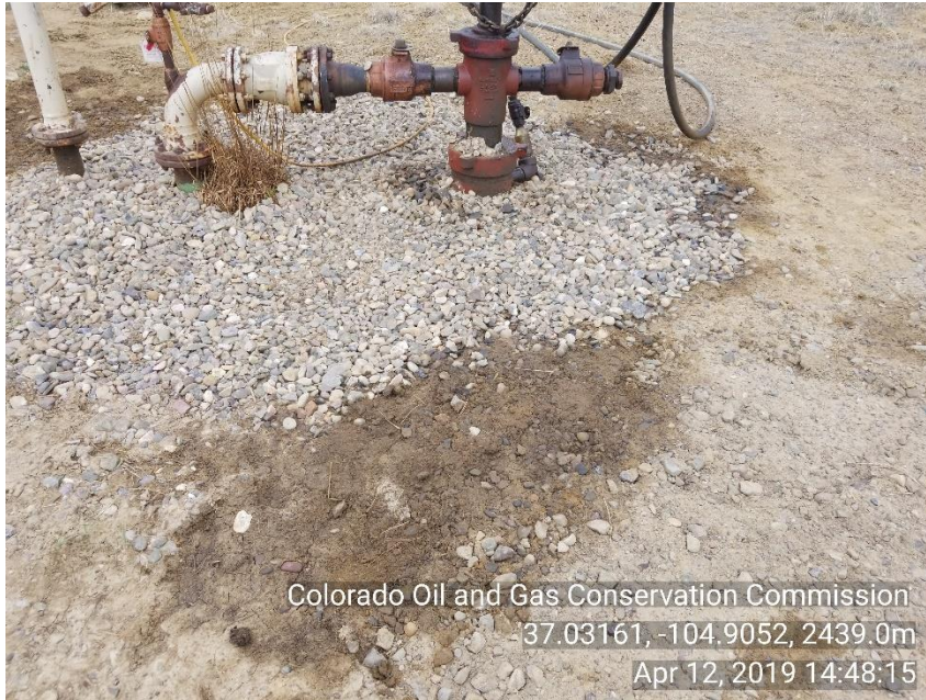
Photo 3 Stained soil; it appears gravel has been placed over stained soil by WH
