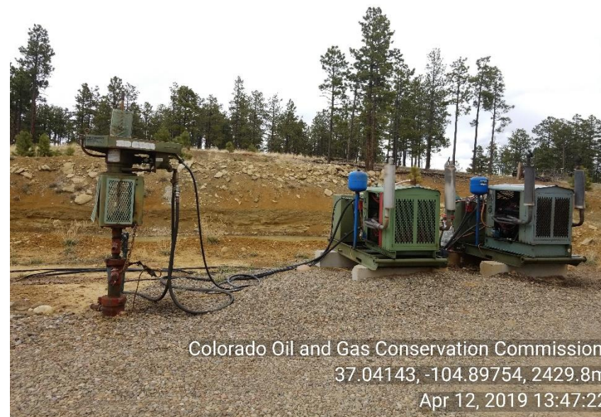
Photo 2 HR#33-06V WH and HYD motor skids for both wells.
