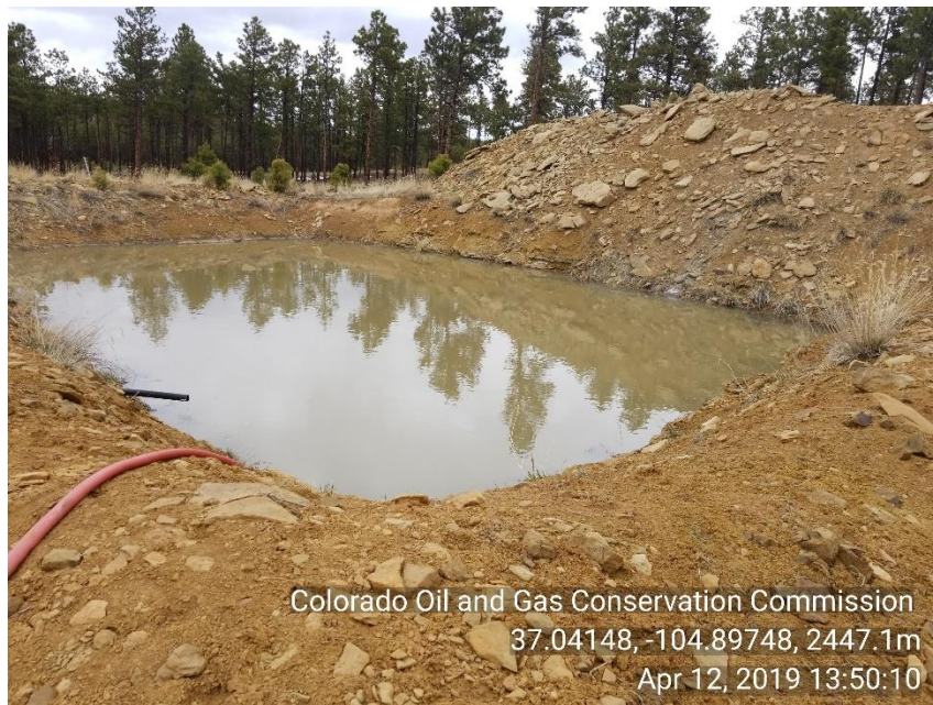
Photo 9 Produced water pit #1
