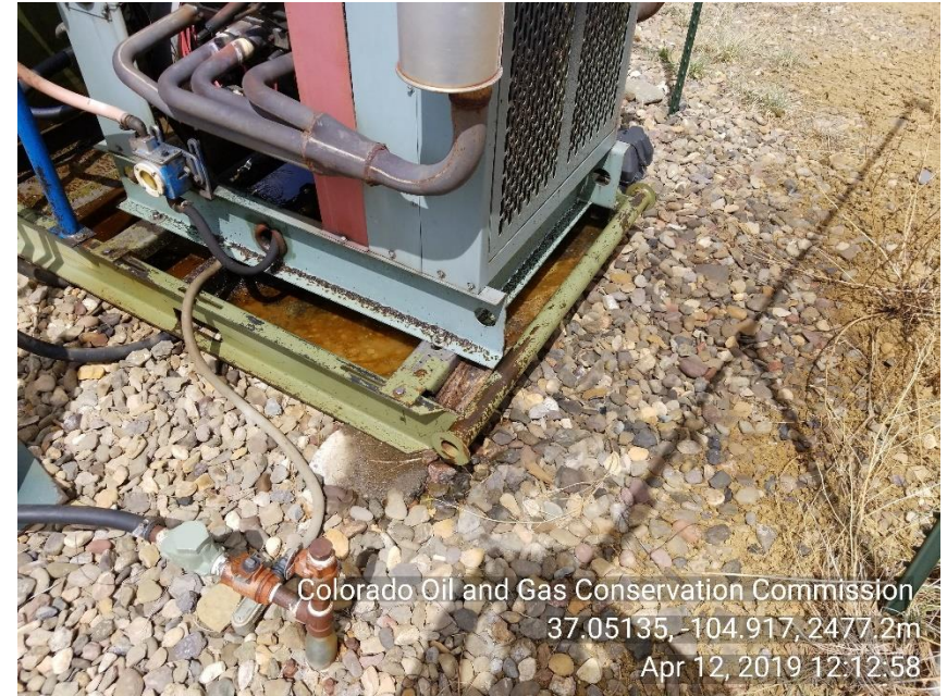
Photo 4 Stained soil around HYD motor skid
