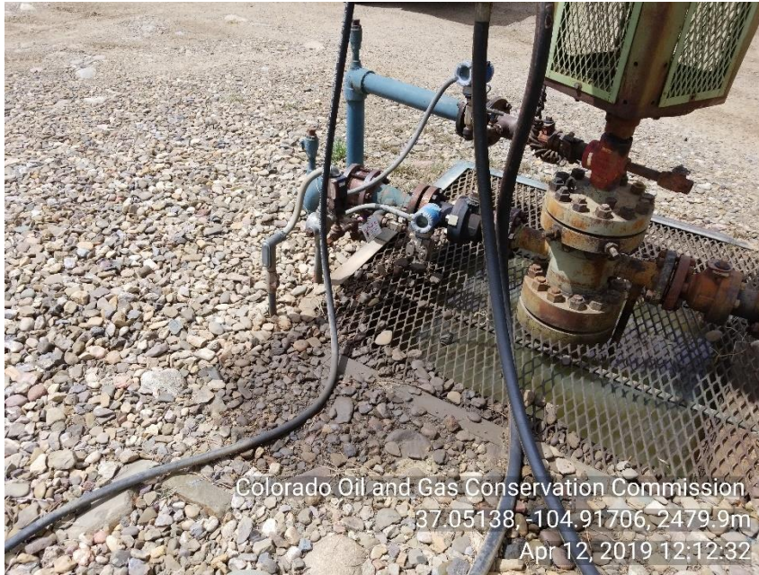
Photo 3 stained soil around WH
