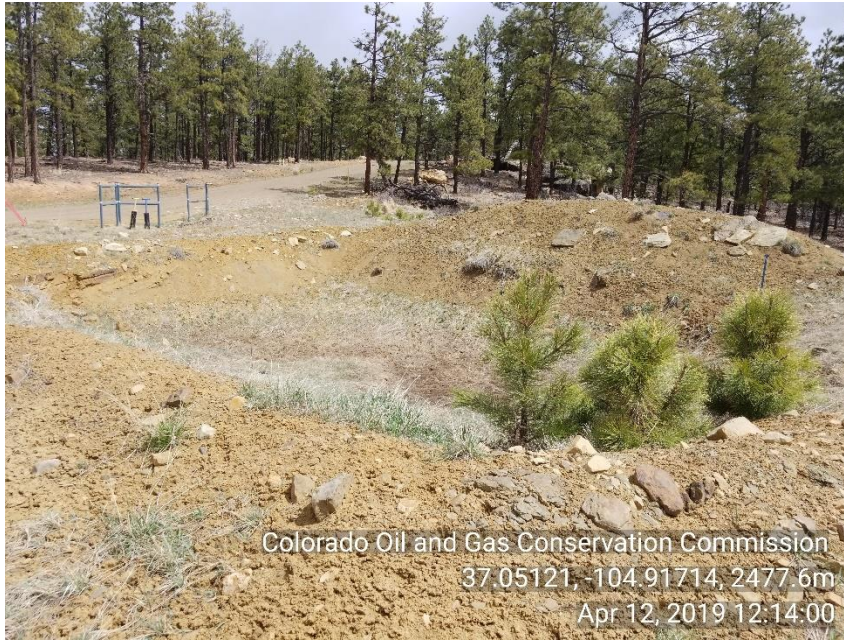
Photo 5 Produced water pit.
