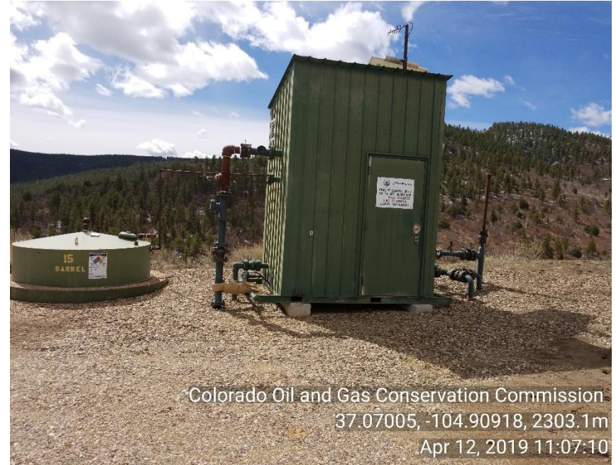
Photo 2 Sep/meter house and 15bbl produced water tank
