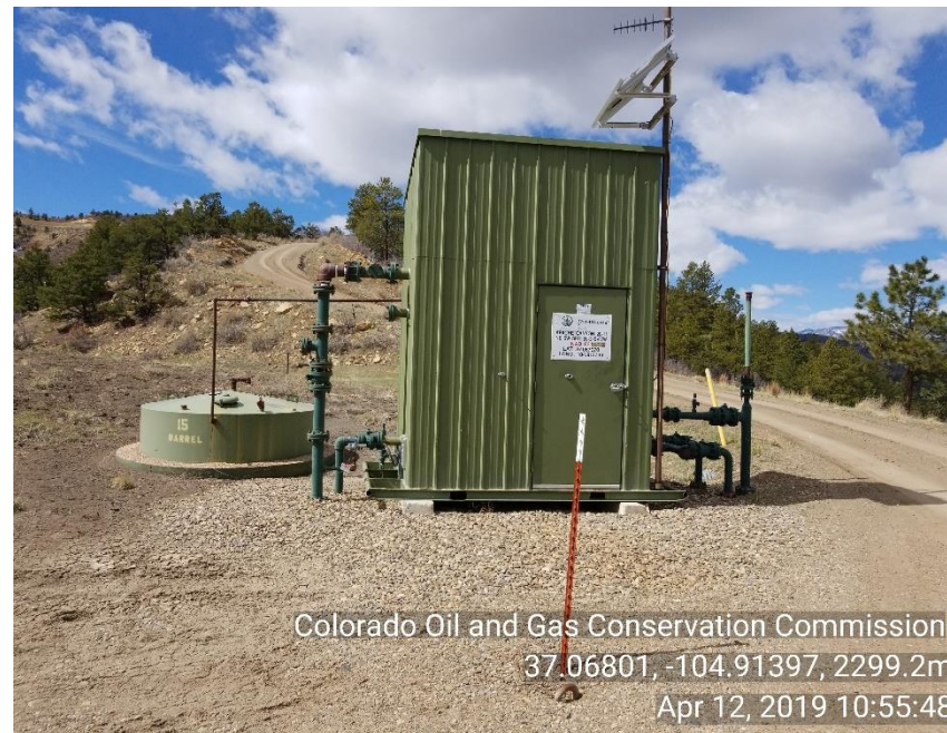
Photo 2 sep/meter house and 15bbl produced water tank.
