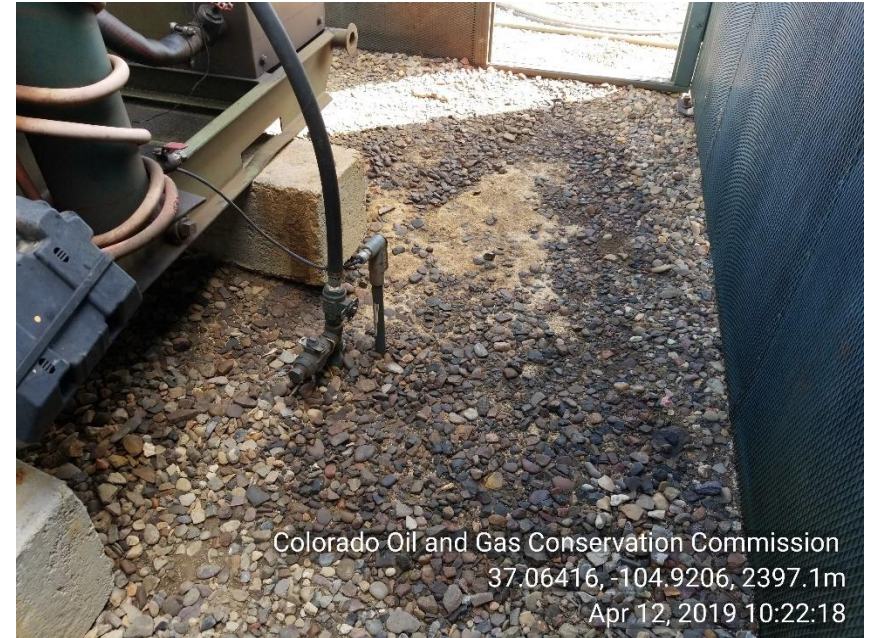
Photo 4 Stained soil around HYD motor skid.
