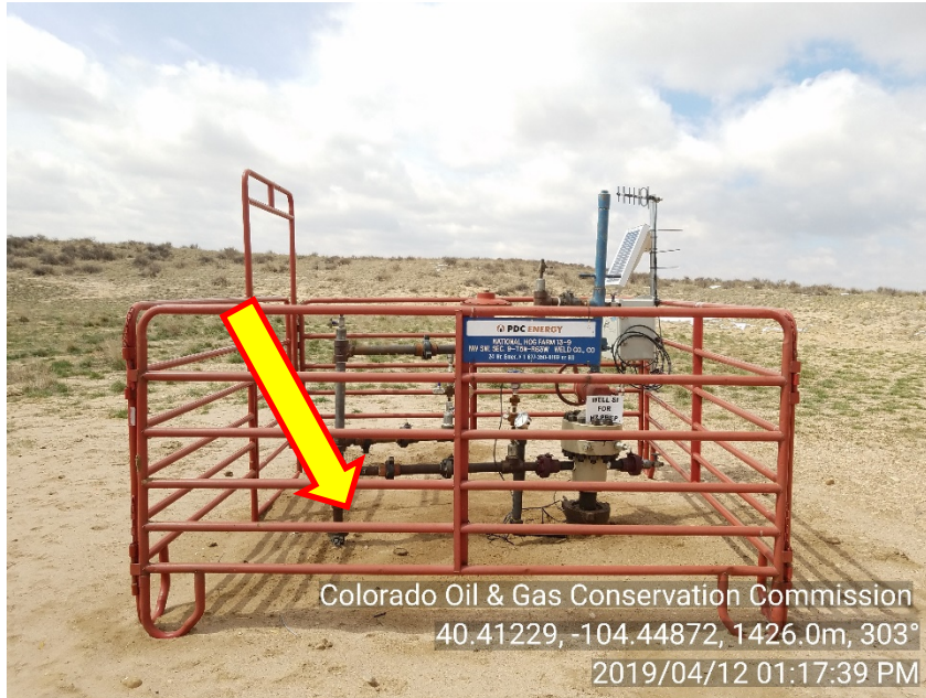
Photo #1 NHF 13-9 (05-123-20921) Wellsite Temporarily Abandoned | TA Stained soil at wellhead perimeter
