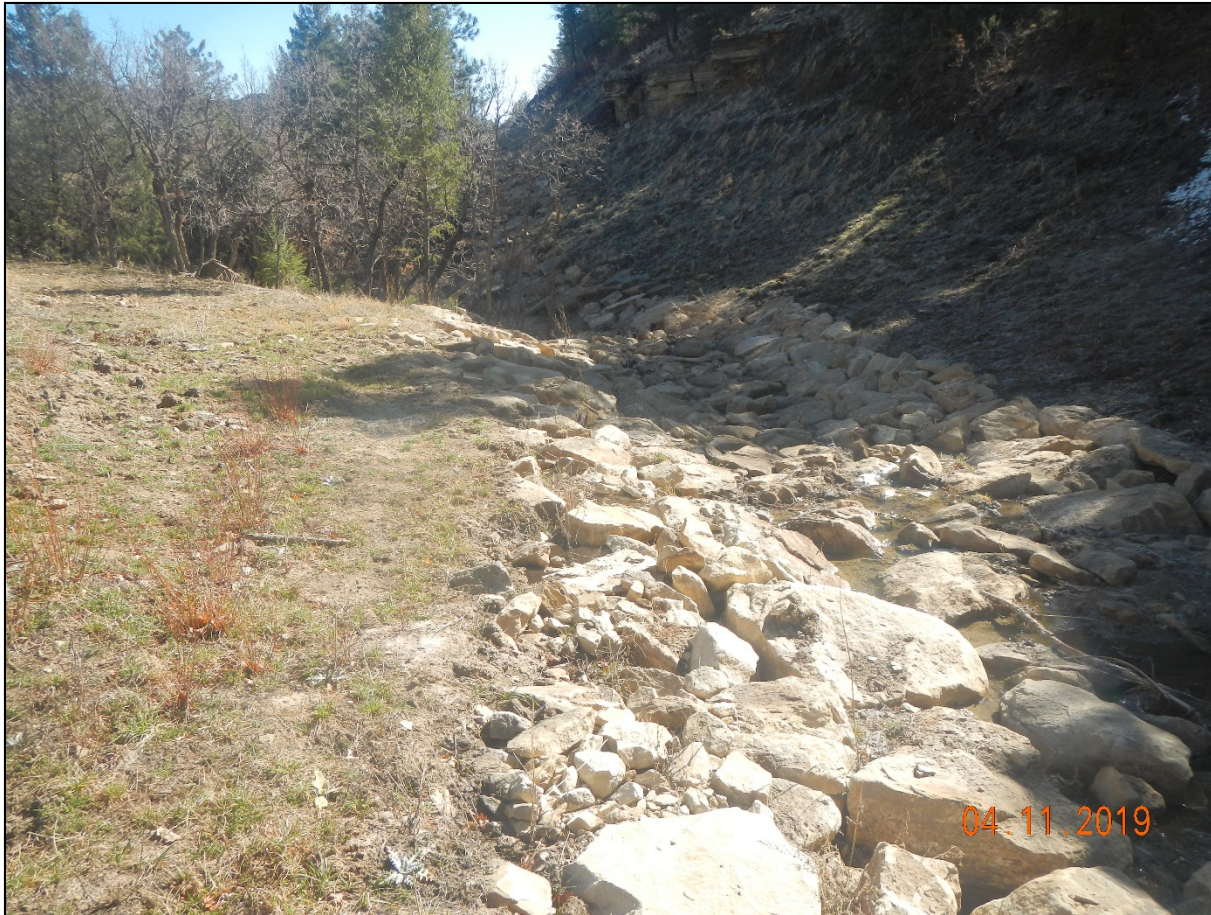
Photo 2. Pipe has been removed from this area. Rock rip/rap has been placed in the drainage for stabilization.
