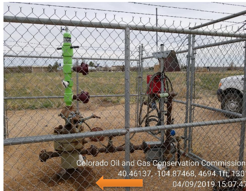
Photo 2 – Casing Collar leak, stained soil
