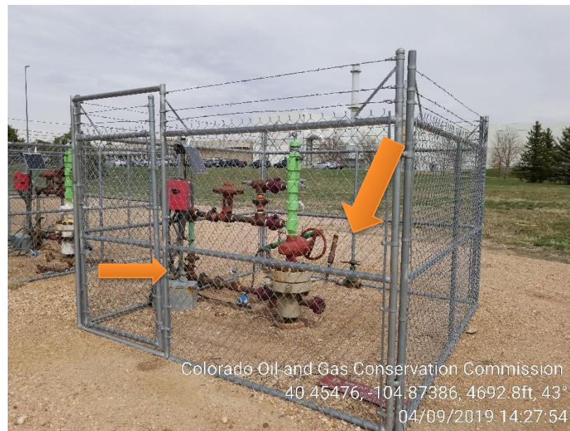
Photo 15 – Well 27-34, unmarked 1" riser, Unused equipment
