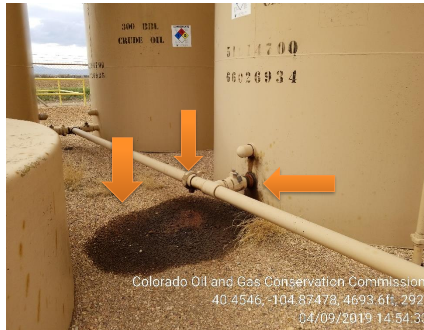
Photo 2 – Stained soil from hammer union
