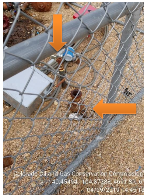
Photo 7 – Well 27-33, unmarked 1" riser, unmarked 2" riser
