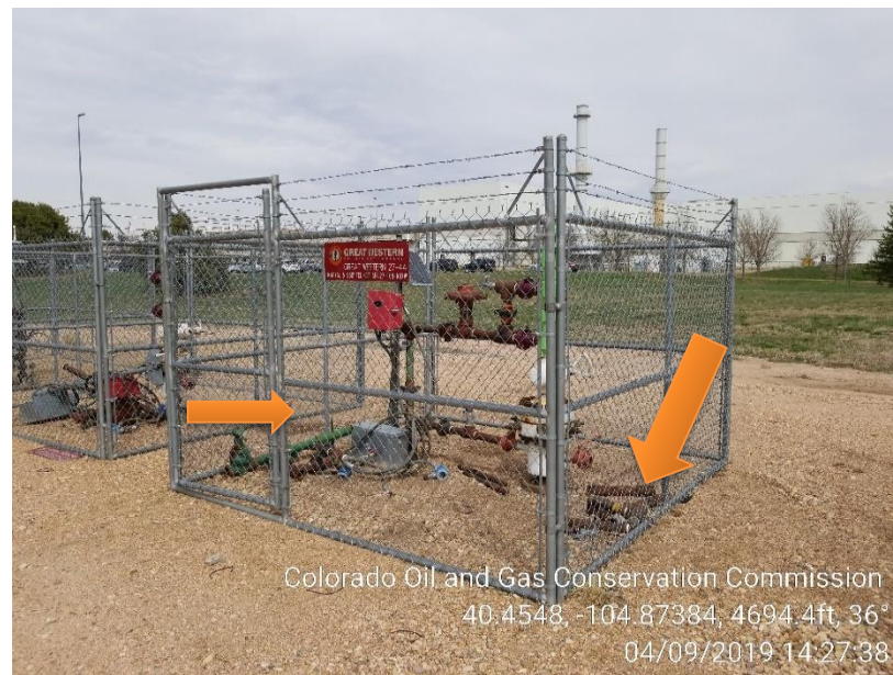
Photo 13 – Well 27-44, unmarked 1" riser, Unused equipment
