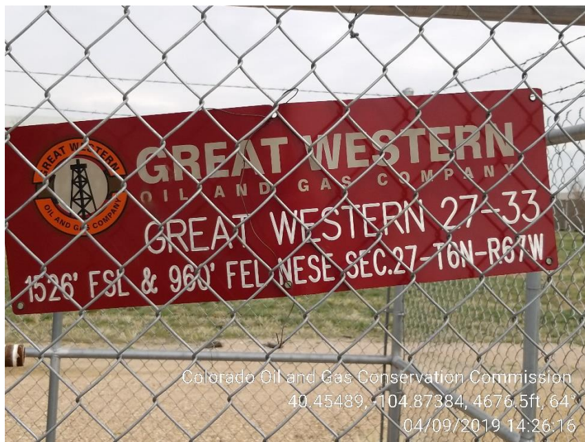
Photo 4 – Wellhead sign for 27-33 missing Emergency Contact info
