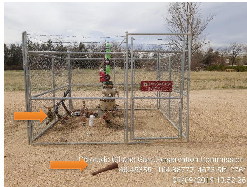
Photo 8 – Wellhead 27-53, TA. Unused equipment
