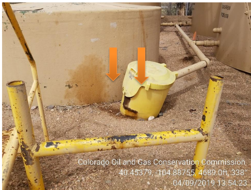
Photo 3 – Stained soil around load line bucket
