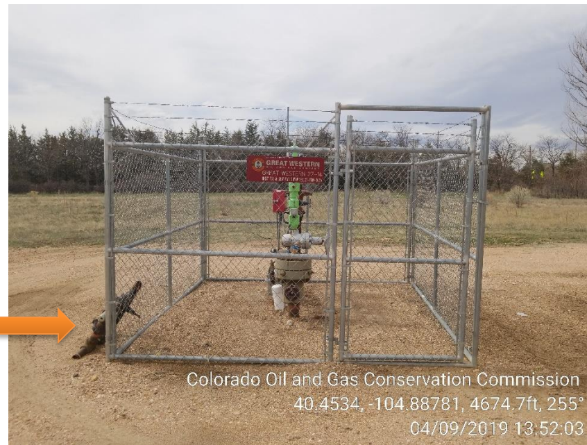
Photo 6 – Wellhead 27-14, Shut-In. Unused equipment
