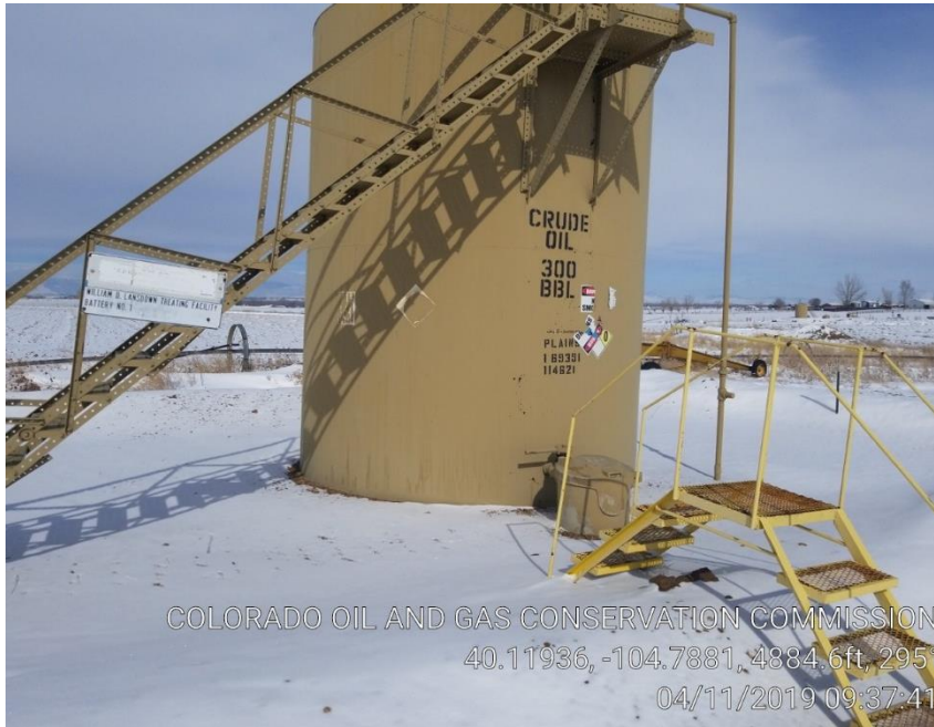
Pic 11 Tank loc sign faded, NFPA placards torn off
