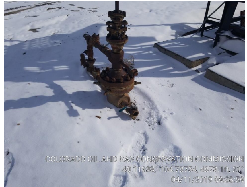
Pic 14 no bull plug installed in production casing valve.
