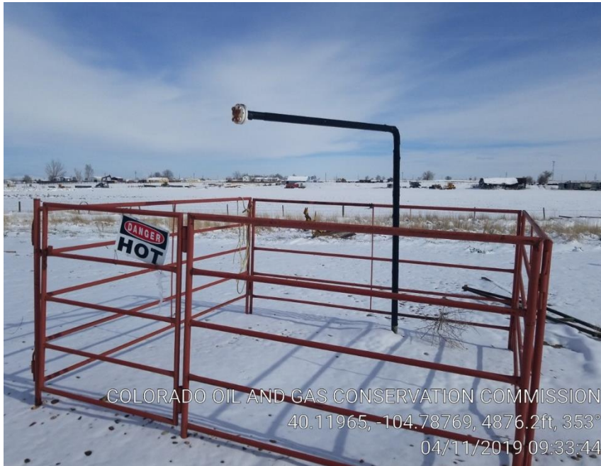
Pic 5 unused unmarked and not LOTO riser
