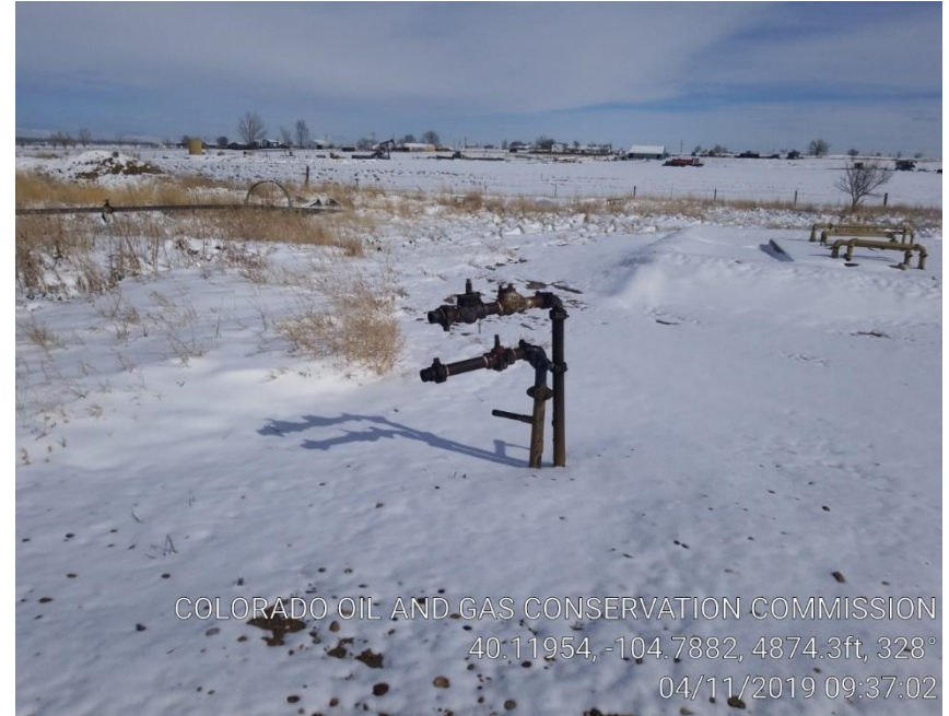
Pic 10 unused unmarked and not LOTO rises, and stained soil.
