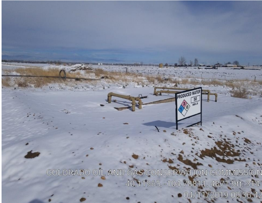
Pic 9 Produced water tank, berms not adequate and in disrepair
