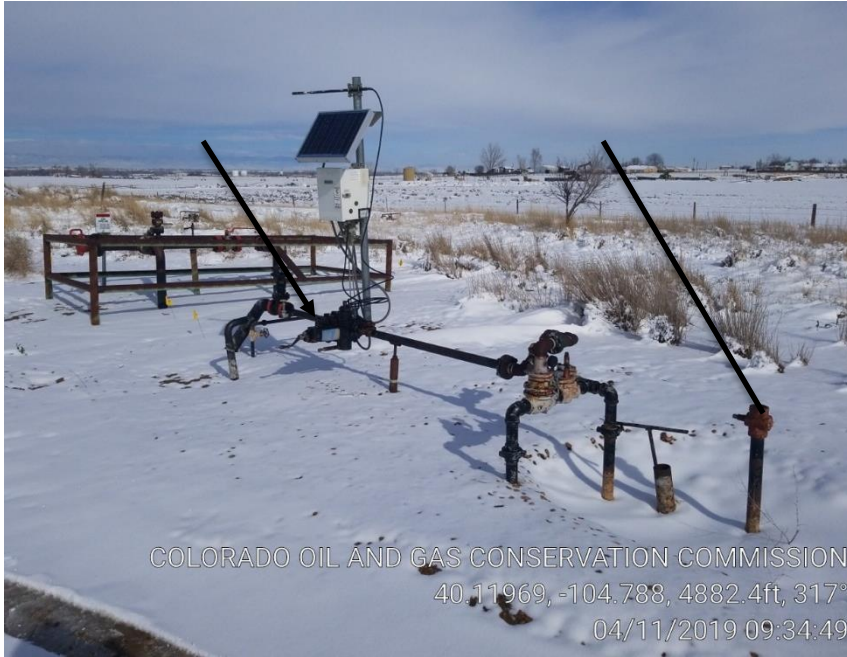
Pic 7 Gas meter run unused. Unmarked and not LOTO risers
