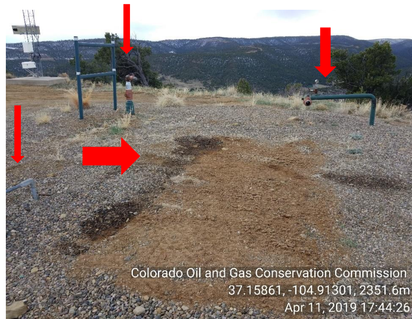
Photo 4 Stained soil and unused, unmarked and not LOTO risers
