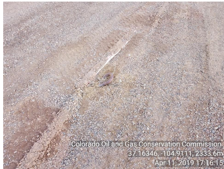
Photo 8 unmarked guy line anchor/
