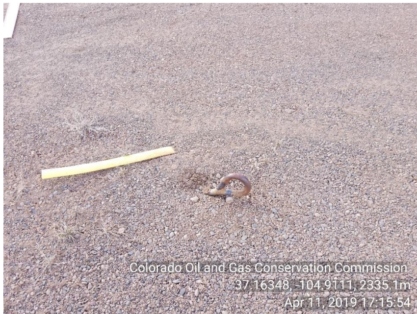
Photo 7 Unmarked guy line anchor.
