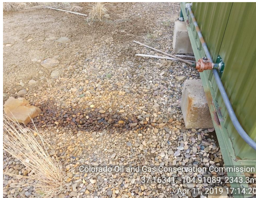
Photo 2 Stained soil under drain line for separator.
