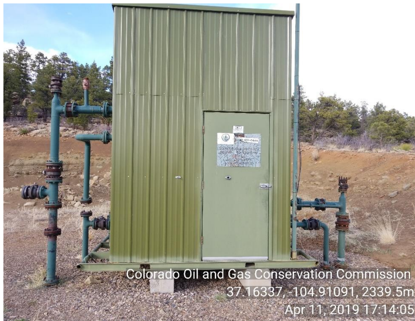
Photo 1 sep/meter house. Location sign is faded and not legible.
