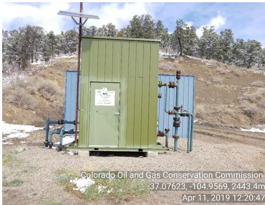
Photo 1 Sep/meter house, Liquid ring sound walls
