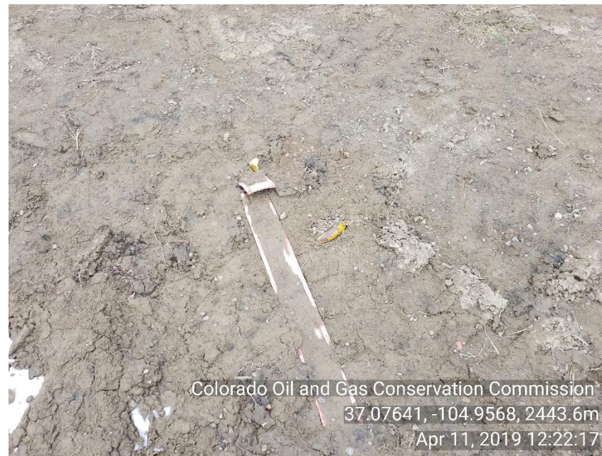
Photo 4 improperly marked guy line anchor
