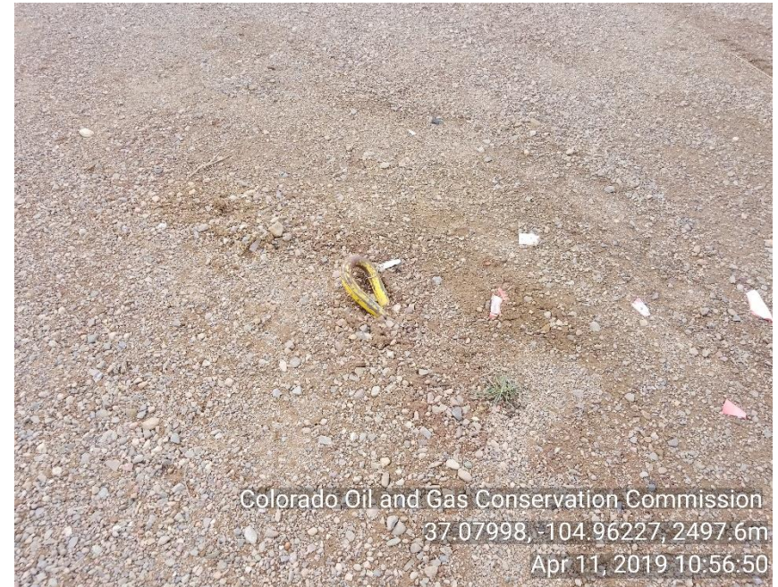
Photo 2 unmarked Guy line anchor
