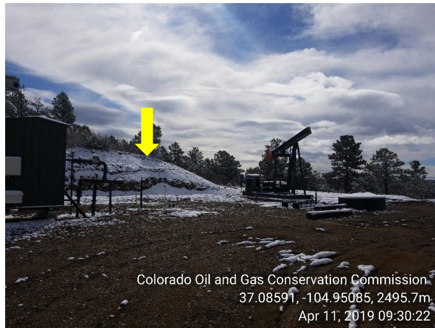
Photo 6 Unmarked, unused and not LOTO riser
