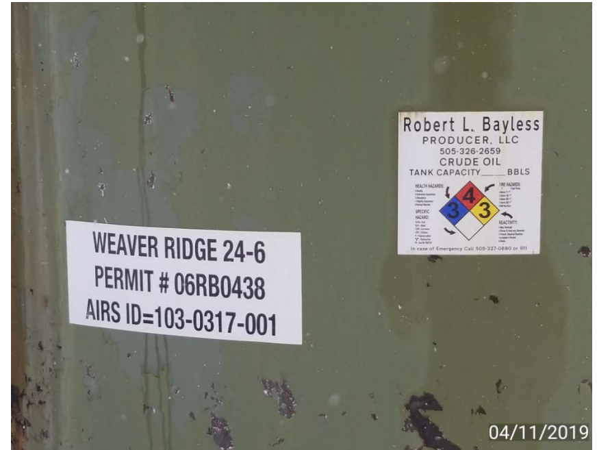
Photo 2. Tank without capacity volume on label.
