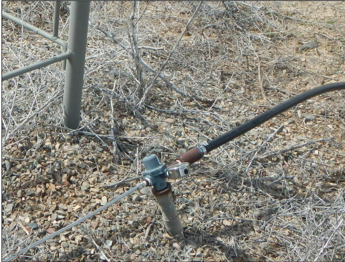
Unmarked unused riser under gas regulator.
