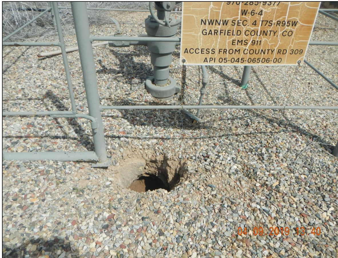
Open hole at gate of well fence.
