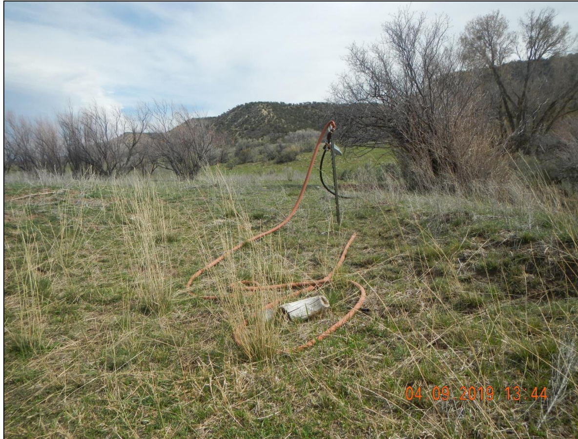
Farm tap supply line and regulator.
