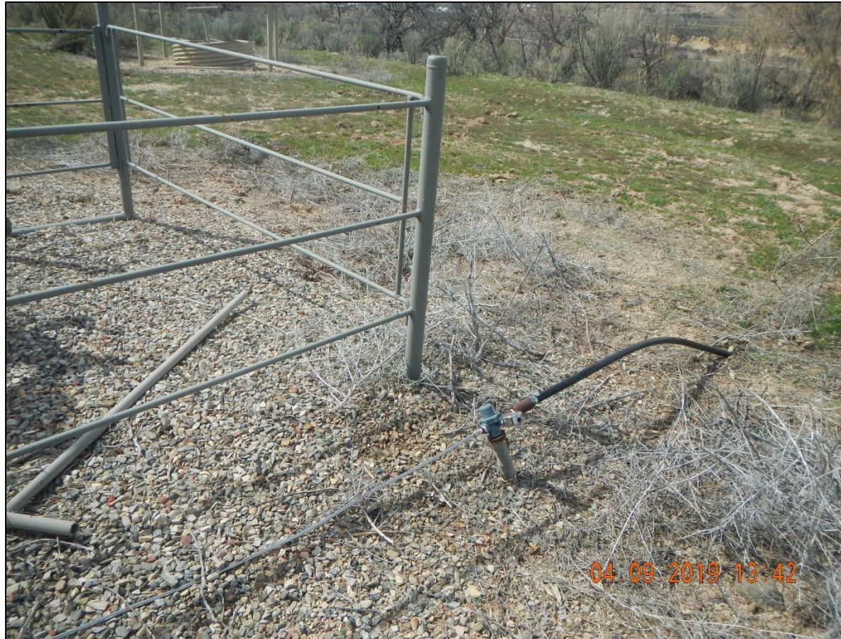
Farm tap line and regulator from well. Unmarked unused riser under gas regulator.
