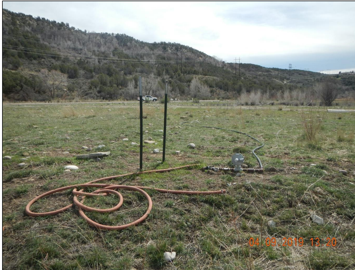
Farm tap: 1- 1" poly pipe connected to PA 342-5 and running off location to a regulator by the pond.
