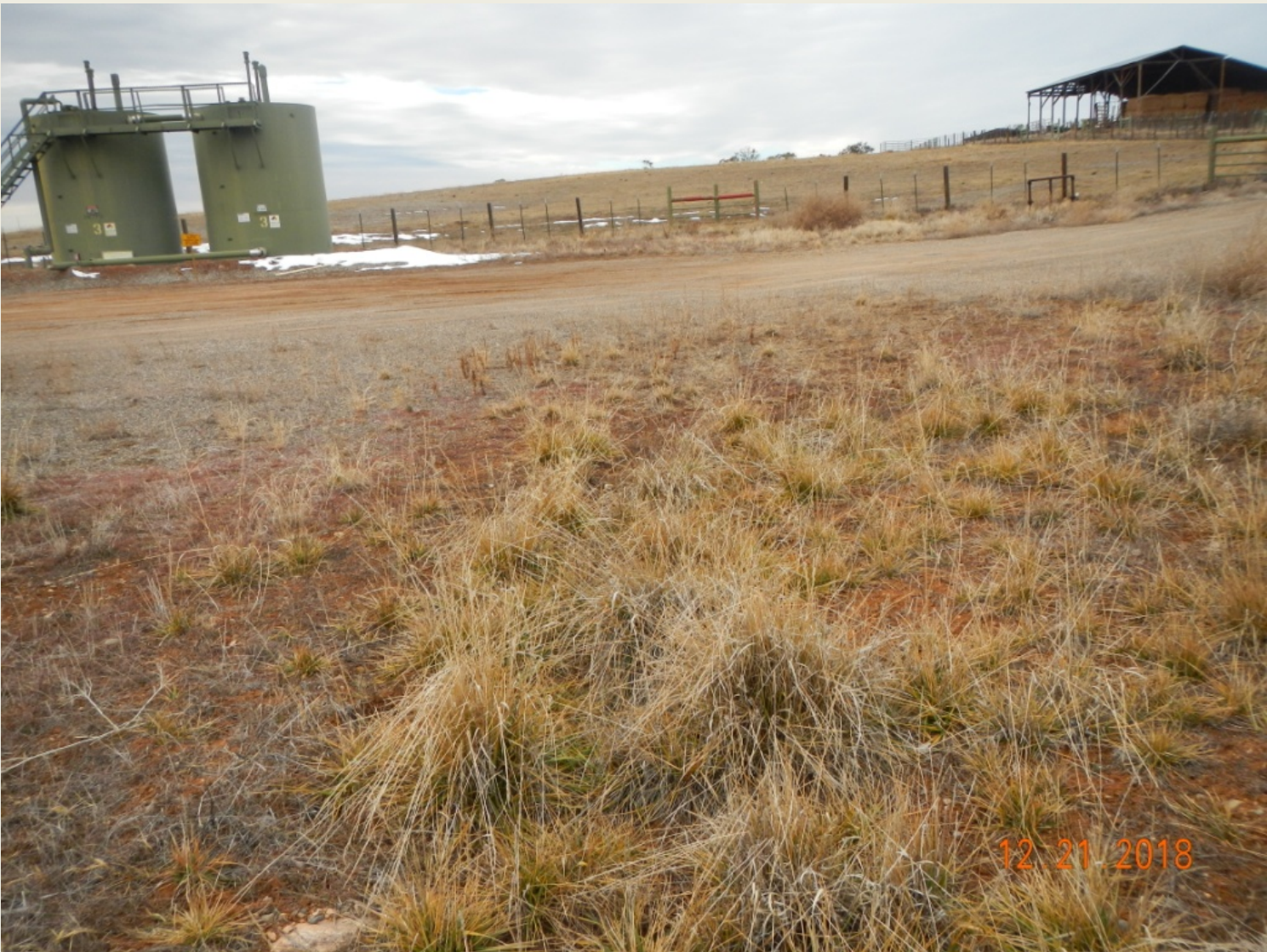
Photo 3. View of the northern project area from the northeastern project area facing westward.
