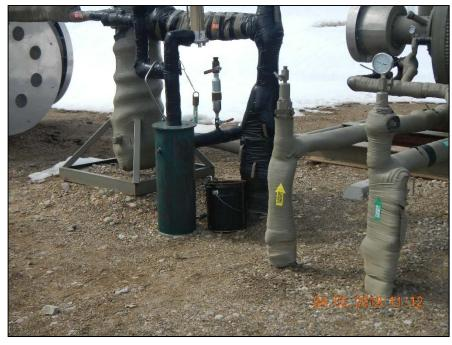
Photo 3. Bucket and stained soil at exhaust.
