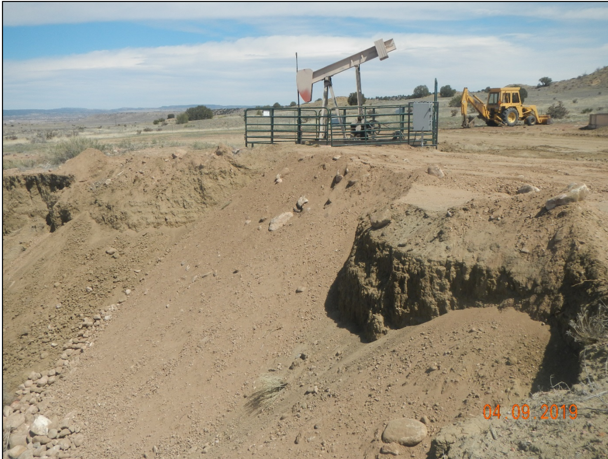
Photo 2. Soil has been brought into the erosional channel near the wellhead. It appears more material is need to slope and stabilize the embankment.
