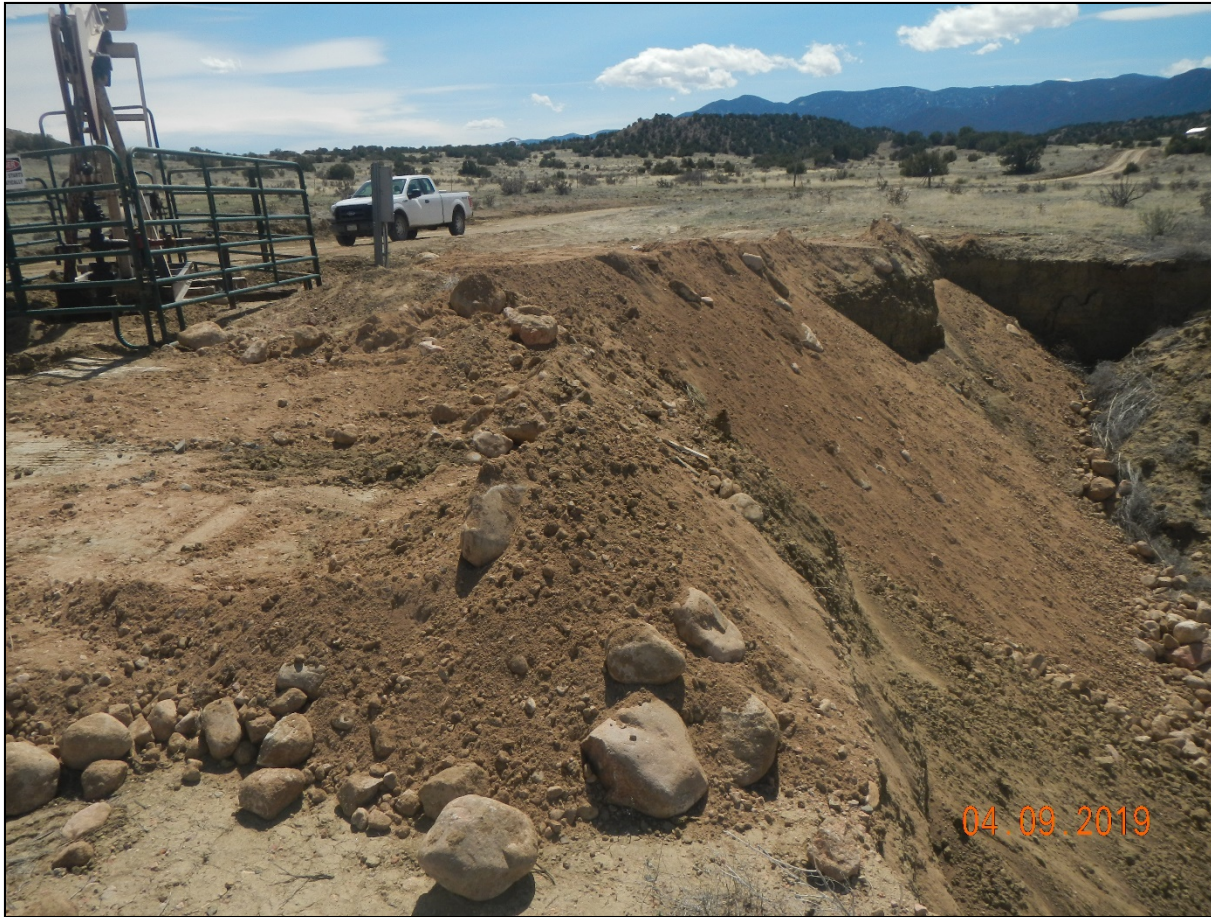
Photo 3. View of the western project area from the western edge facing southward. Wellhead is adjacent to an erosion channel. This area needs immediate stabilization to prevent any further erosion.
