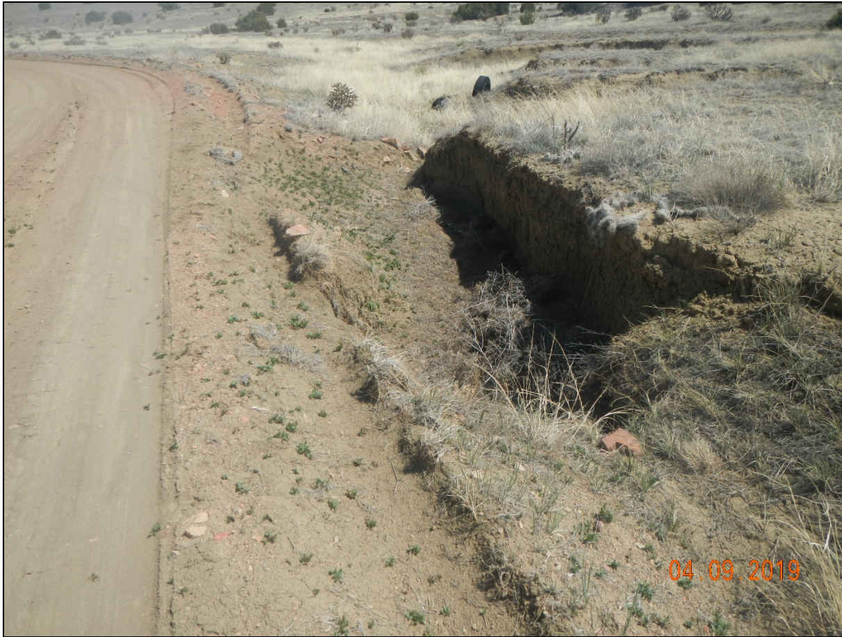
Photo 5. View of erosional headcut, approximately 3 feet wide and deep, along the access road (Lat/Long:38.33276,-105.11330. Stormwater controls have not been installed.
