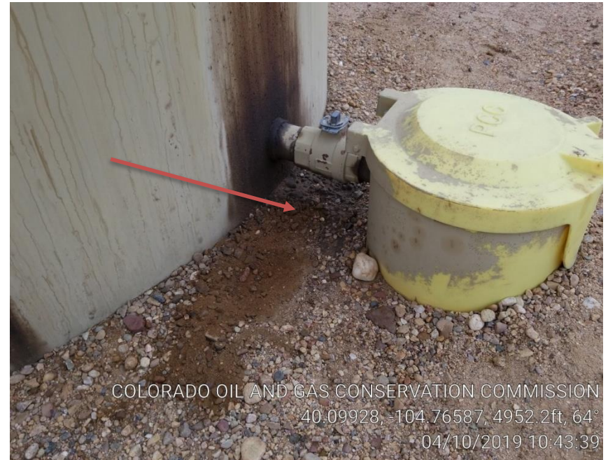
Pic 6 possible leak on back of oil tank.
