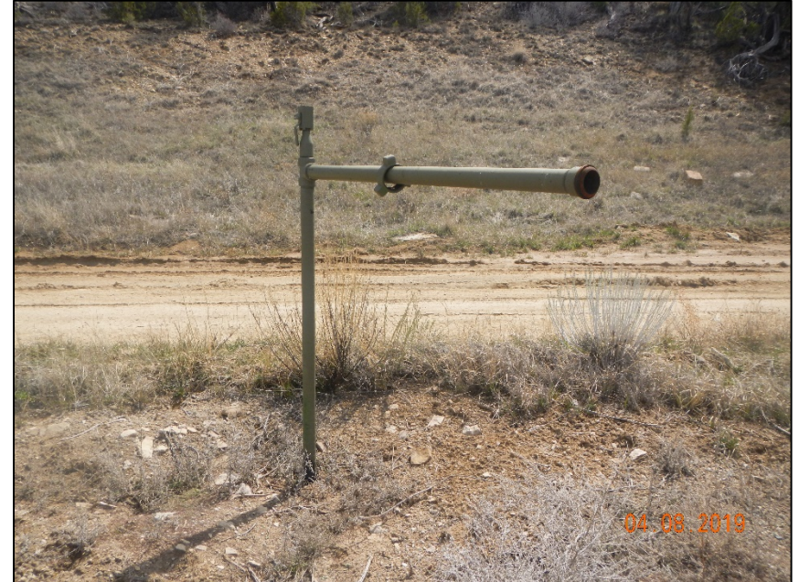
Riser unmarked and untagged on location
