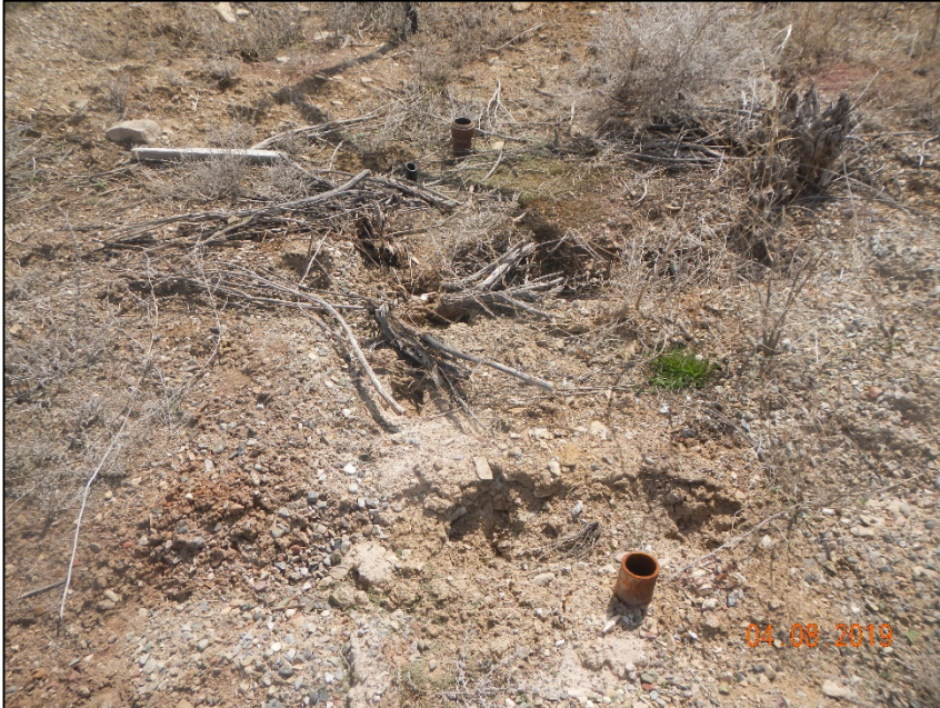
Riser unmarked and untagged on location
