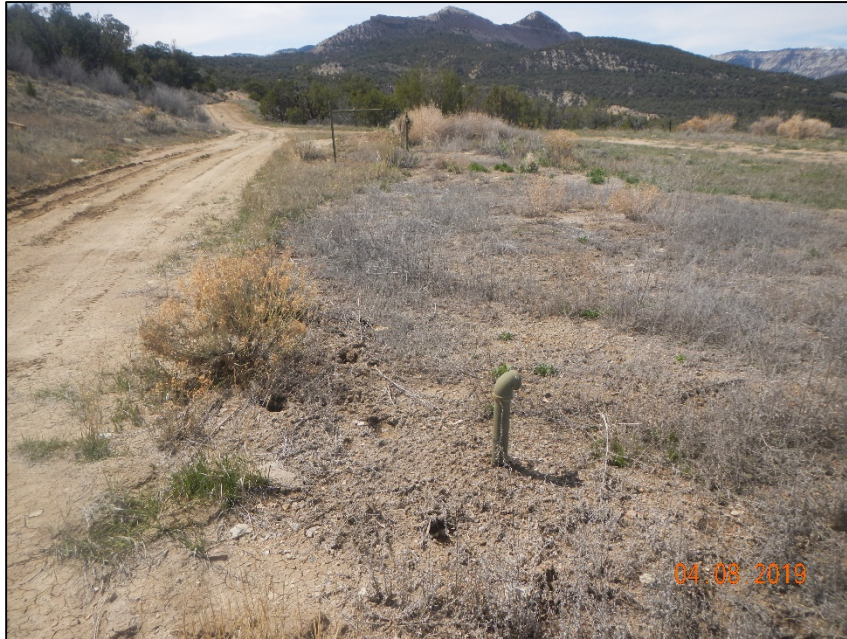
Photo #2. Riser unmarked and untagged on location
