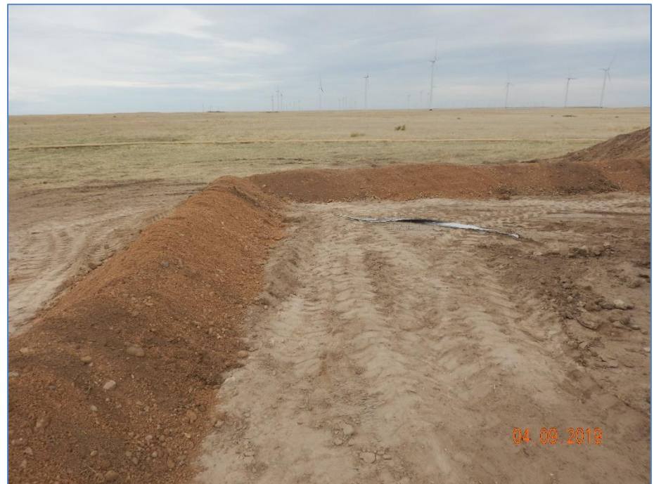
Photo 4: Photo taken from the red tank, facing east. Photo taken during a follow-up visit later in the day. Photo shows soils were returned to the stockpile and that the berms constructed and in proper functioning condition.
