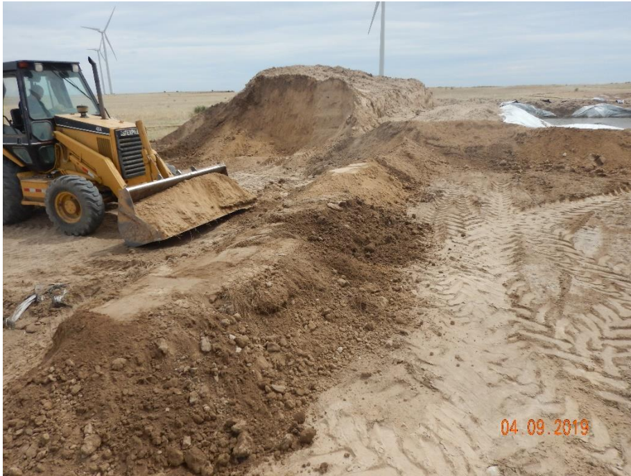
Photo 1: Photo taken from the east end of the location, facing south. Photo shows contractor on site was utilizing the soil stockpile salvaged from the pit, as material for the berms around the tank. Inspector discussed concerns regarding 1002.c with Mr. Dick Shanor who was also on location at time.
