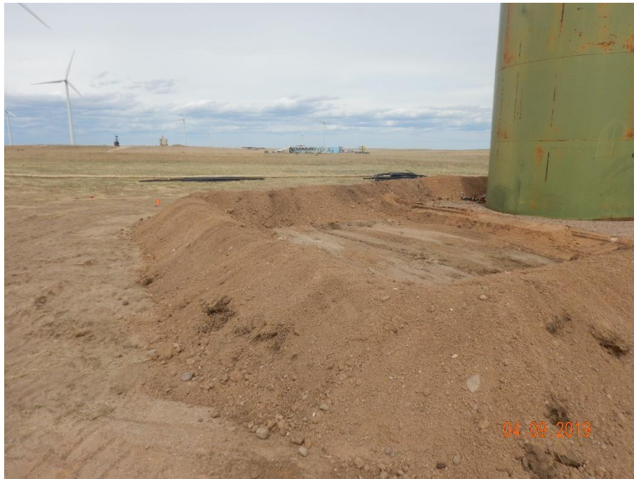
Photo 3: Photo taken from the southwest corner of the tank battery. Photo shows operator has updated the secondary containment.
