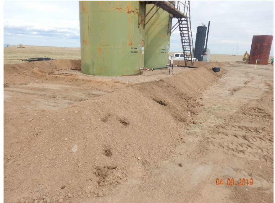
Photo 2: Photo taken from the southwest corner of the tank battery. Photo shows operator has updated the secondary containment.
