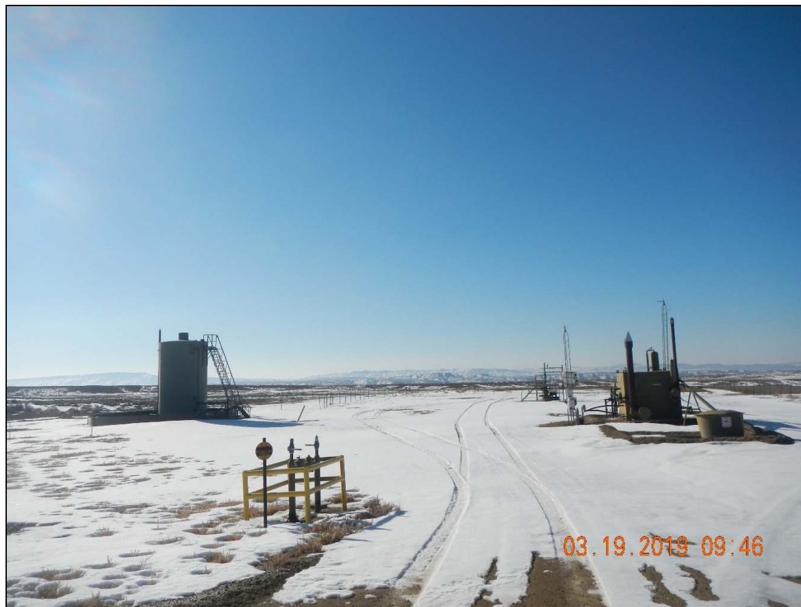
Photo 1. Overview of location taken at entrance facing northwest.
