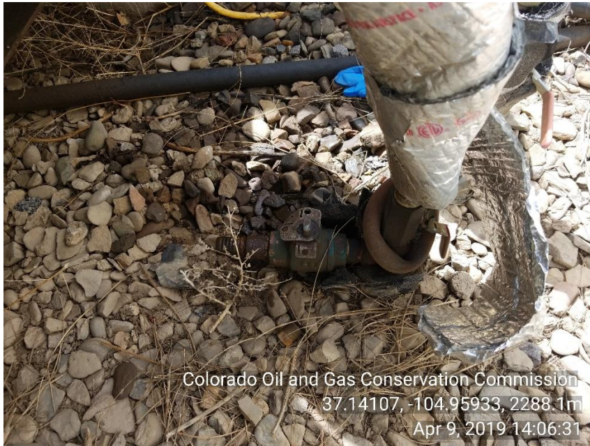
Photo 3 Stained soil around fuel gas line to HYD skid
