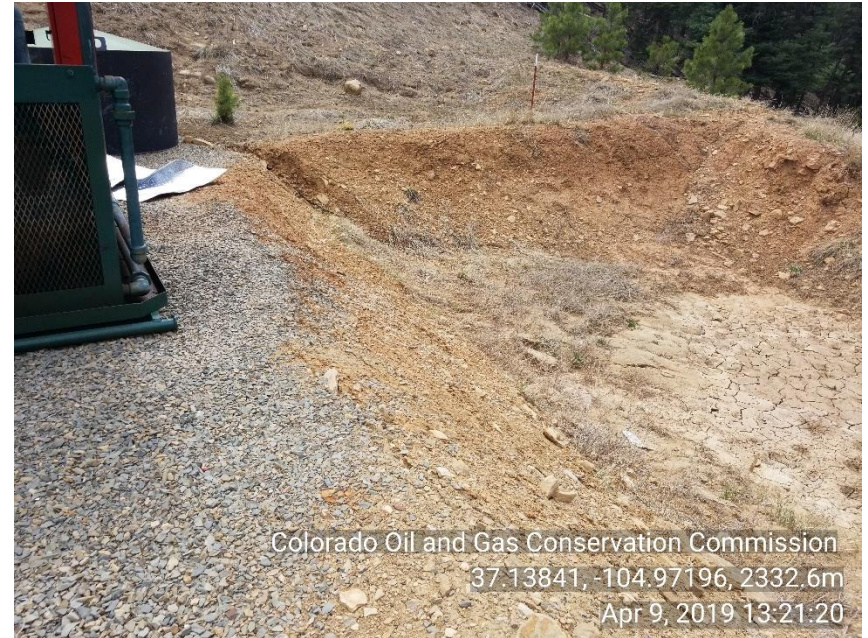
Photo 8 Storm water no berm around back side of production pit
