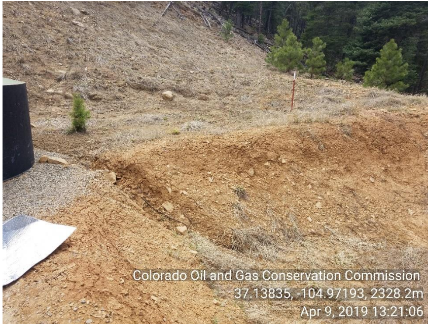
Photo 7 storm water erosion from back of location making large reel into produced water pit
