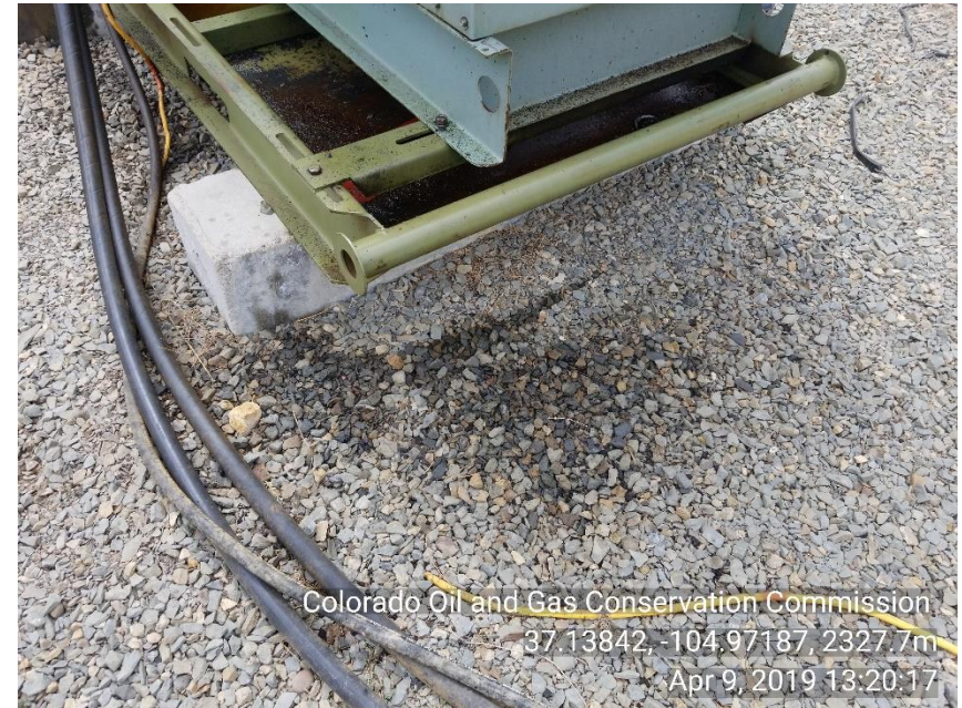
Photo 4 Stained soil around HYD skid
