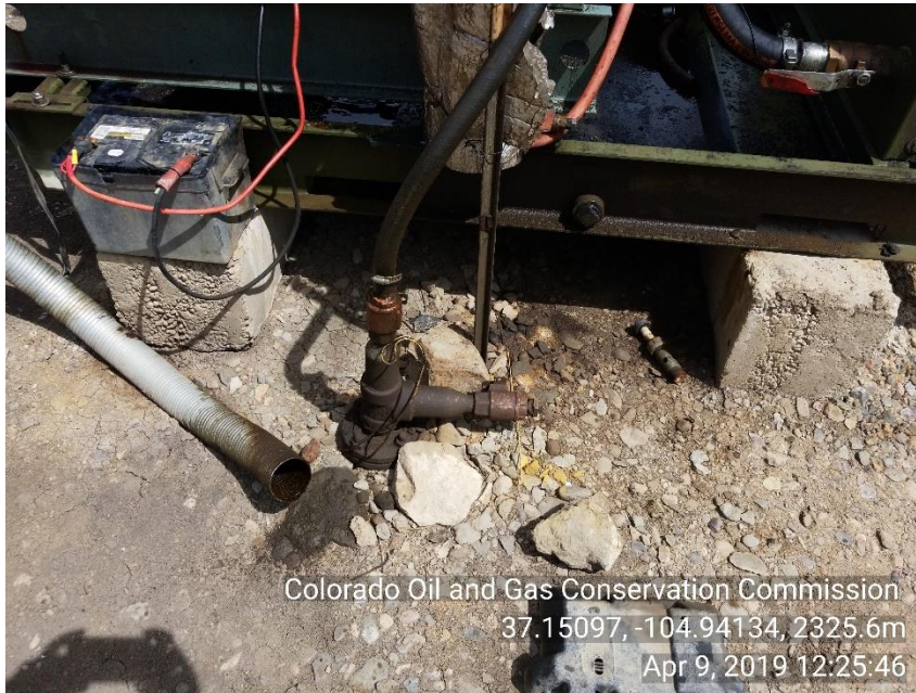
Photo 5 Stained soil around HYD skid
