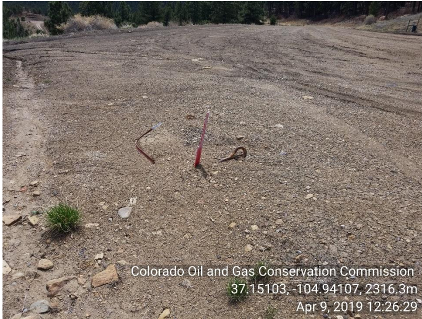
Photo 7 Guy line anchor not properly marked
