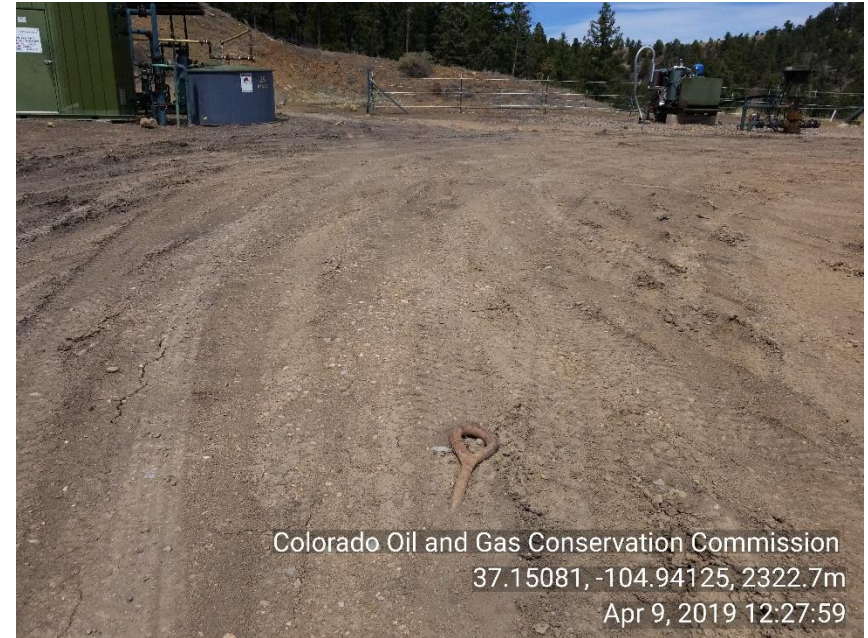
Photo 8 Guy line anchor marker missing
