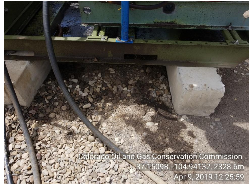
Photo 6 Stained soil around HYD skid
