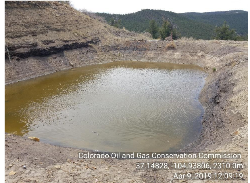
Photo 4 Produced water pit
