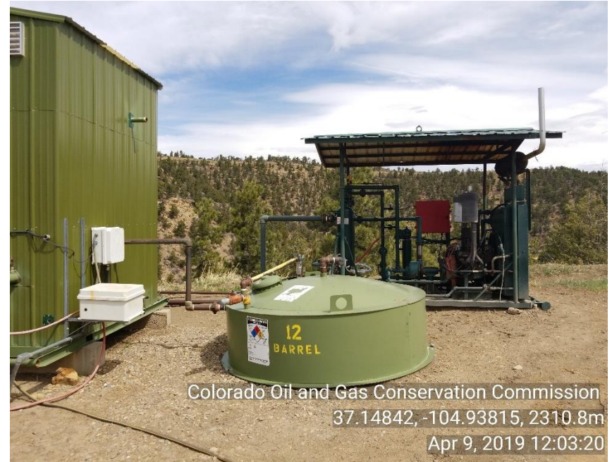
Photo 2 liquid ring and produced water tank
