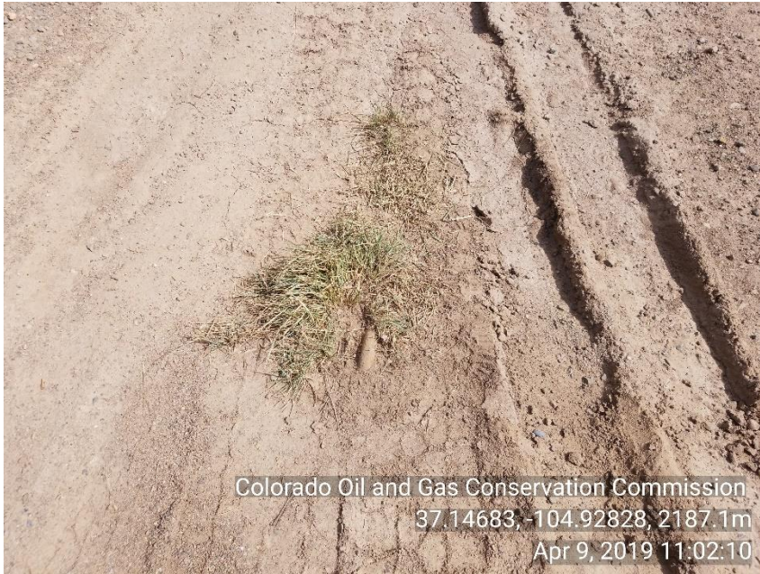
Photo 11 Unmarked Guy line anchor
