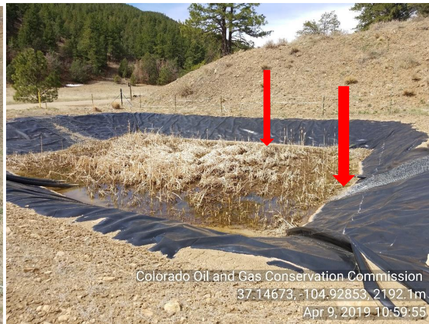
Photo 10 storm water: pit appears to have sediment and growth in liner.
