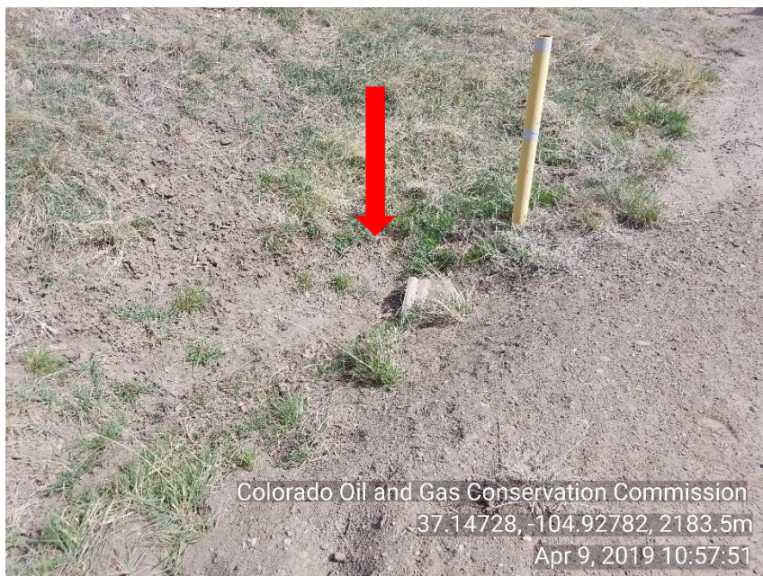
Photo 5 Culvert at entrance to location plugged allowing storm water and sediment to flow across access road in to water way.
