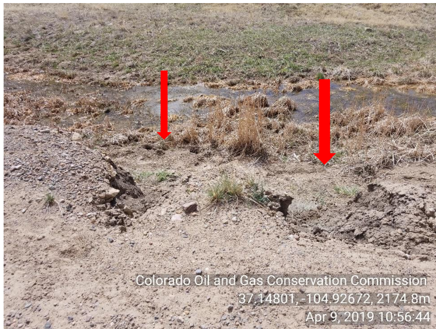
Photo 3 Storm water: Reels on road to location allowing sediment into water way
