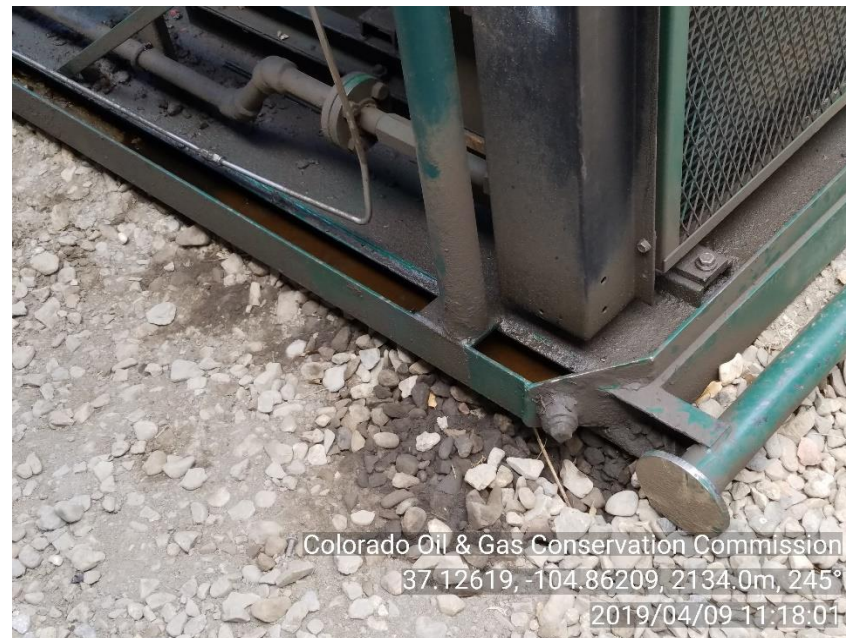
PHOTO 4: IMPACTED SOIL ON EAST SIDE OF COMPRESSOR SKID NEAR SKID DRAIN PLUG.
