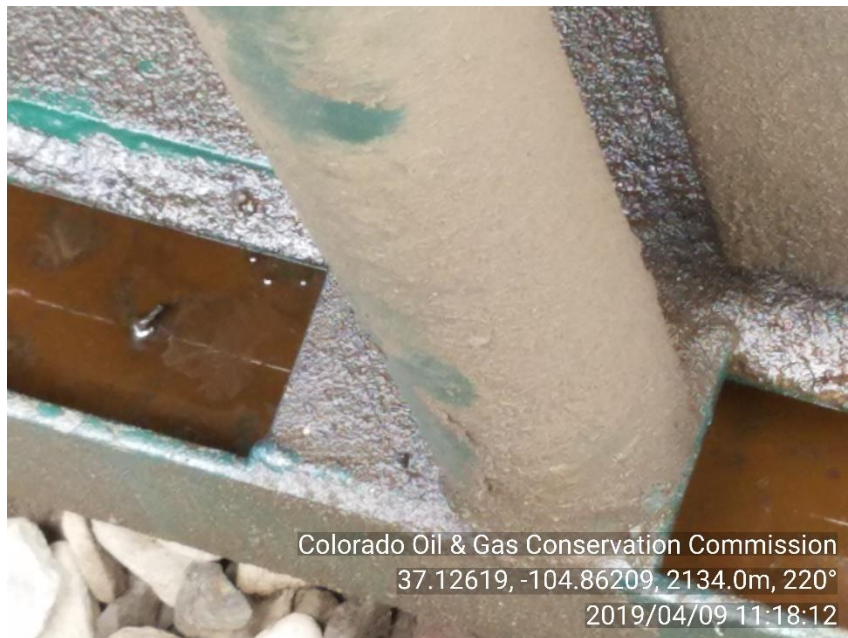
PHOTO 3: COMPRESSOR SKID HAS ROUGHLY 1.5 INCHES OF OIL.
